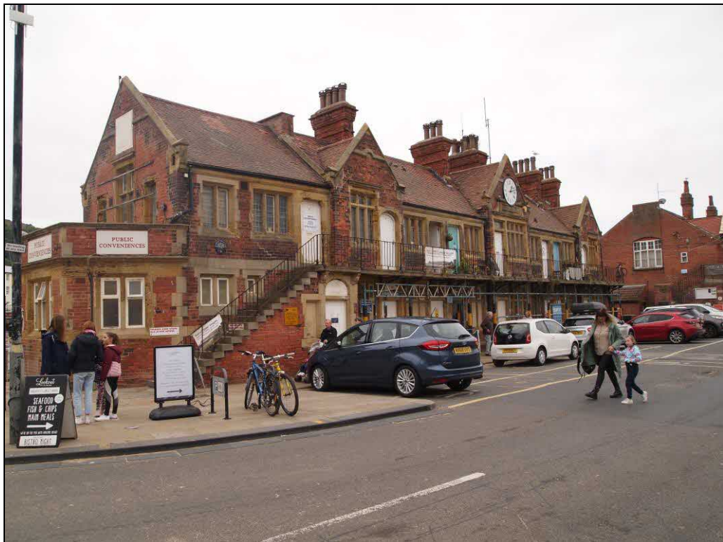
Figure 5: Building 1 front elevation.
