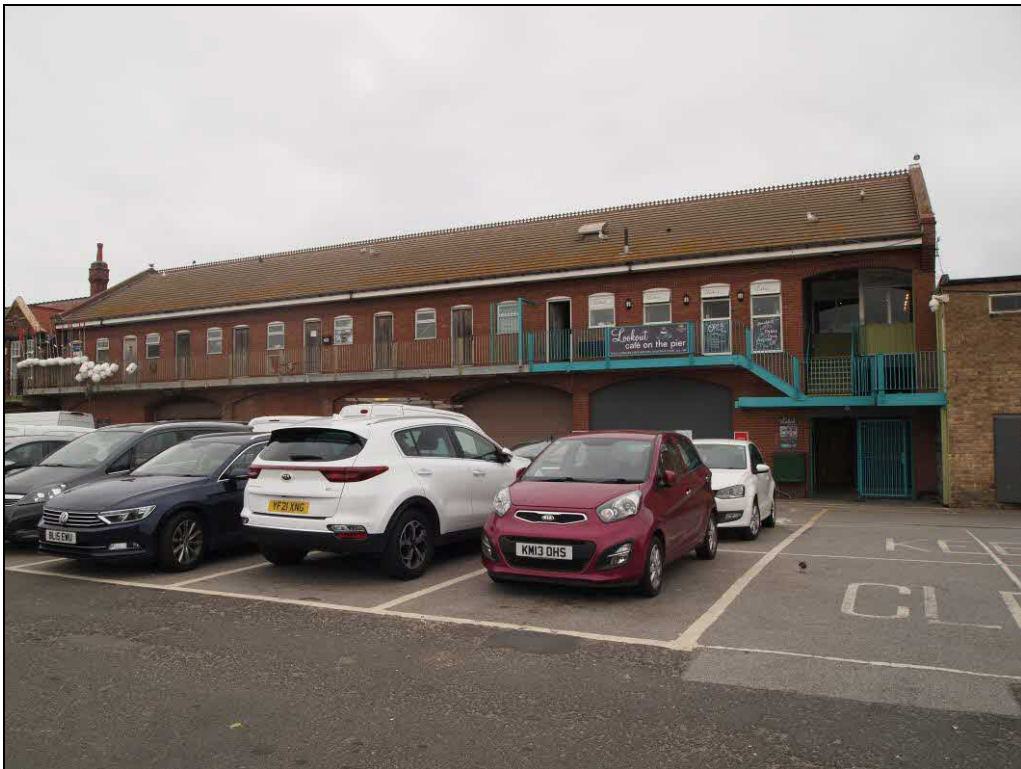
Figure 11: Building 3 front elevation.
