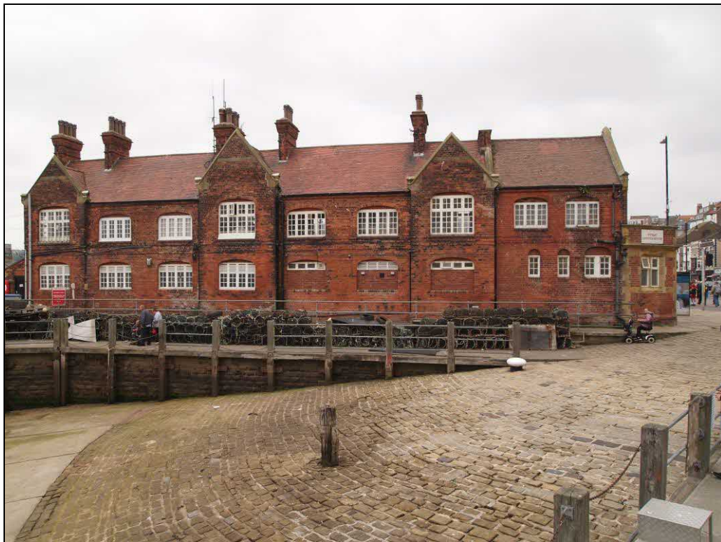
Figure 6: Building 1 rear elevation.
