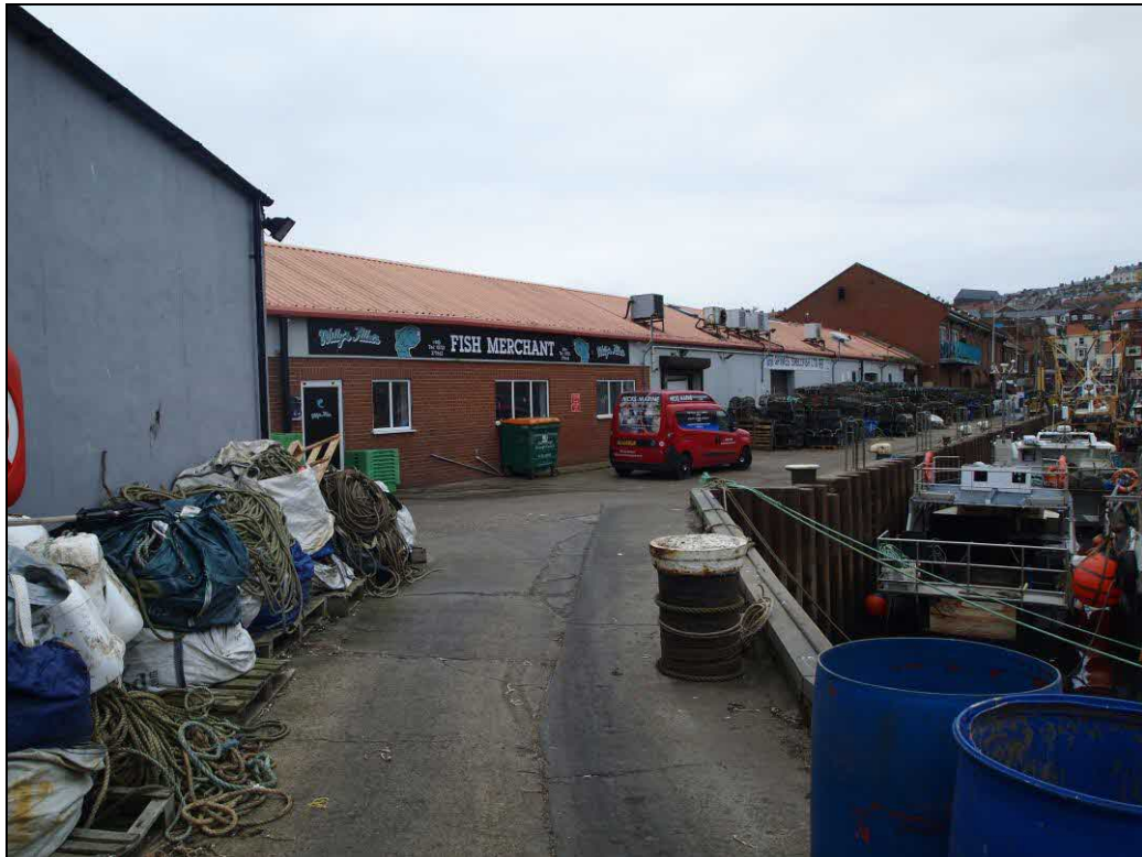
Figure 12: Building 4 rear elevation.
