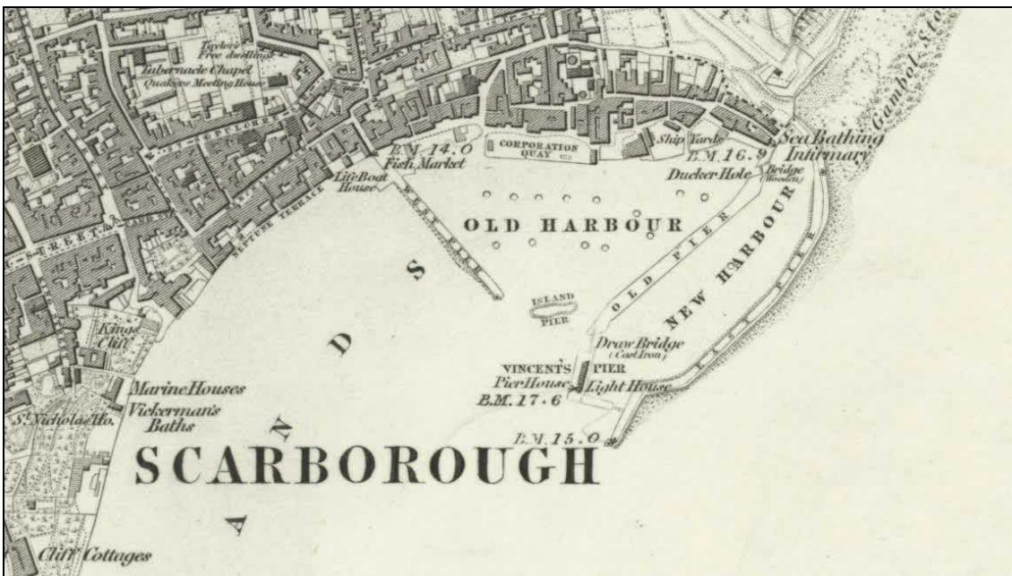
1850 – West Pier in its original form as constructed in 1817.
