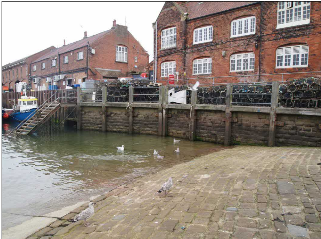
Figure 3: Sandstone wall possibly from original pier structure built in 1817.
