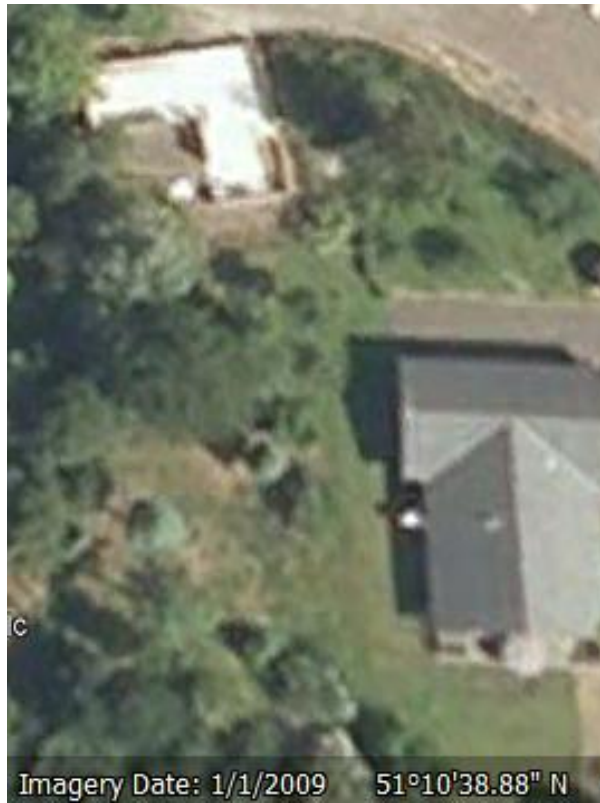
Aerial image showing stables under construction 1/1/2009
