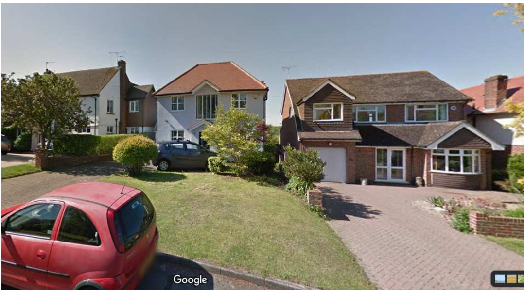
Streetview: Houses 40, 38 and 36
