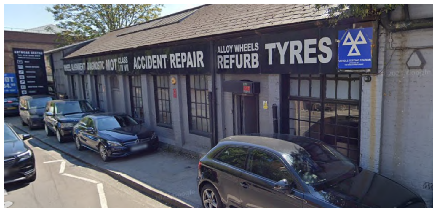
400 Bollo Ln. Facing site to the South.
