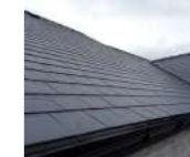
Slate Roof Tiles
