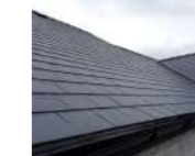
Slate Roof Tiles
