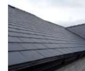
Slate Roof Tiles
