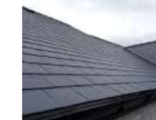
Slate Roof Tiles
