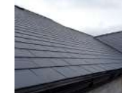
Slate Roof Tiles
