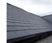
Slate Roof Tiles
