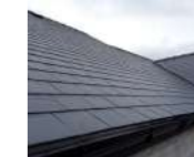
Slate Roof Tiles
