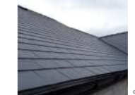
Slate Roof Tiles
