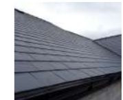
Slate Roof Tiles
