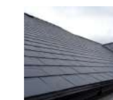
Slate Roof Tiles
