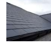
Slate Roof Tiles
