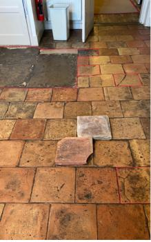
These photographs highlight the typical condition of existing kitchen pamments that would be considered for replacement (with red line boundary). The random placement of flagstones (partly visible in the left-hand photo) will be rationalised and focused to an area in front of the range. Areas of cement flooring (to the left-hand side of the range) will be removed, and replaced with reclaimed pamments.
