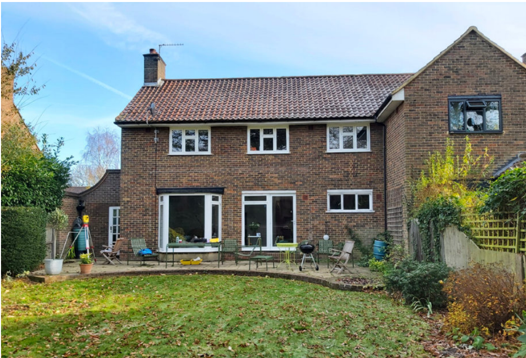
BELOW: View of the existing rear elevation to 11 Allison Grove and part neighbouring property no. 9 Allison Grove to the right (South).
