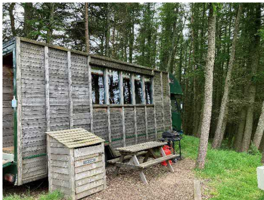
Photograph 3: Timber clad Horsebox (in retrospect)
