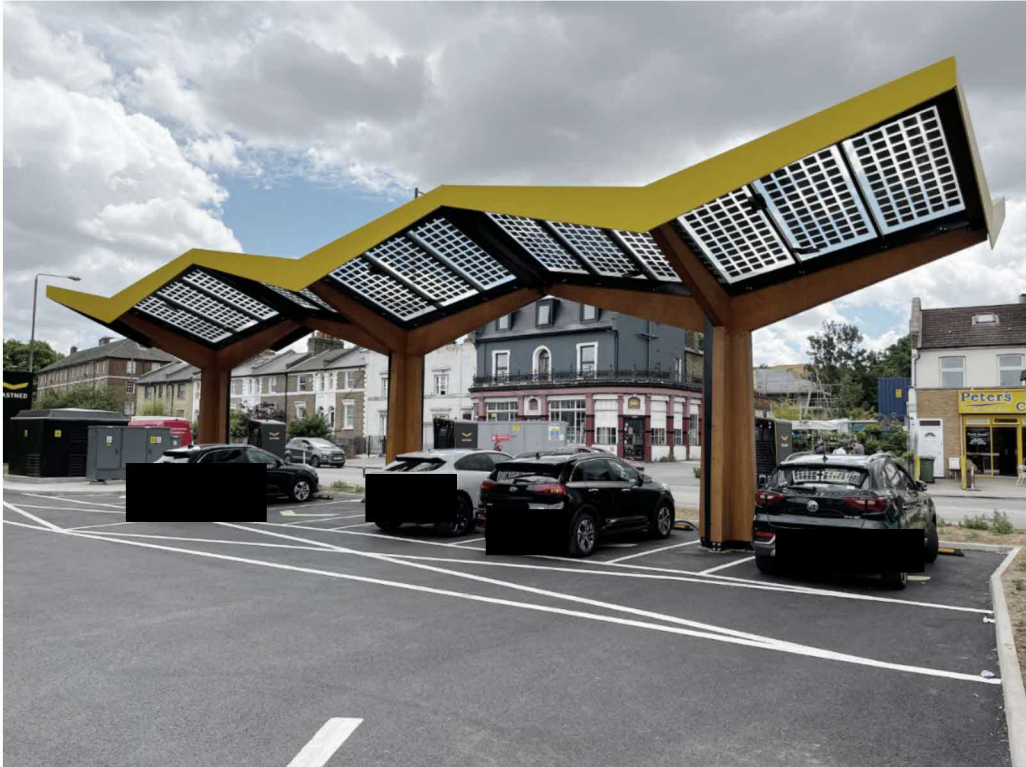
Figure 2.7 A recently completed charging station at Ramac Way in Greenwich, London.
