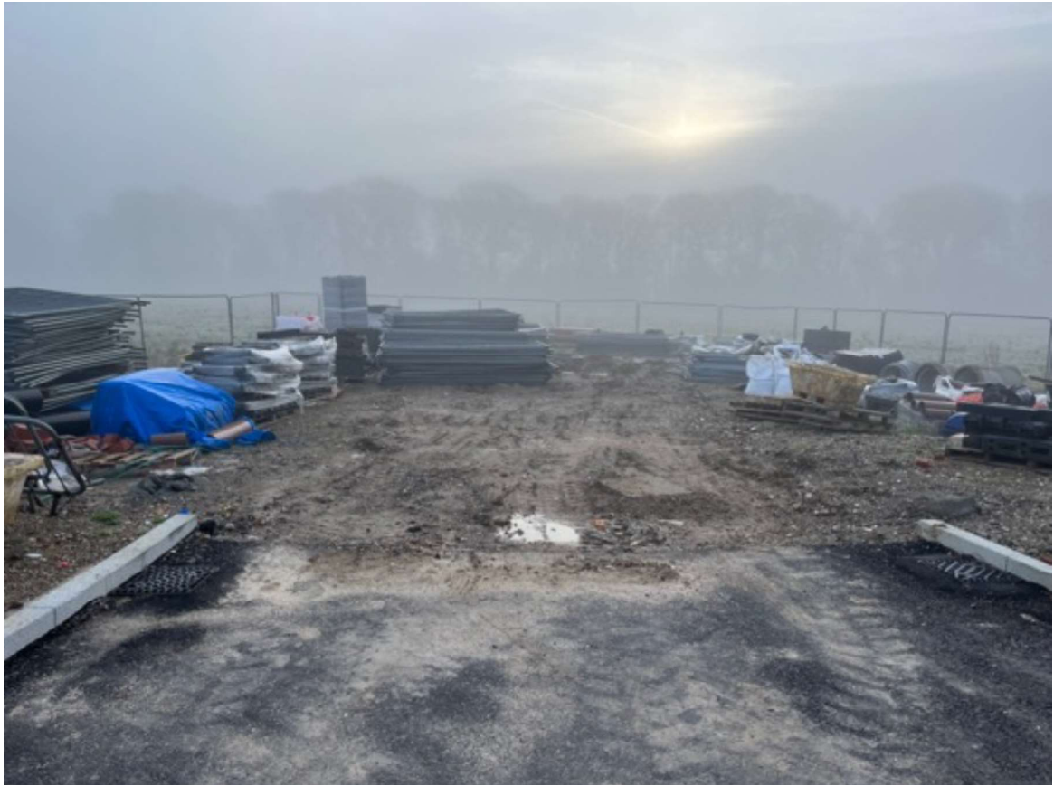
Photo 3: Location of proposed temporary construction compound.
