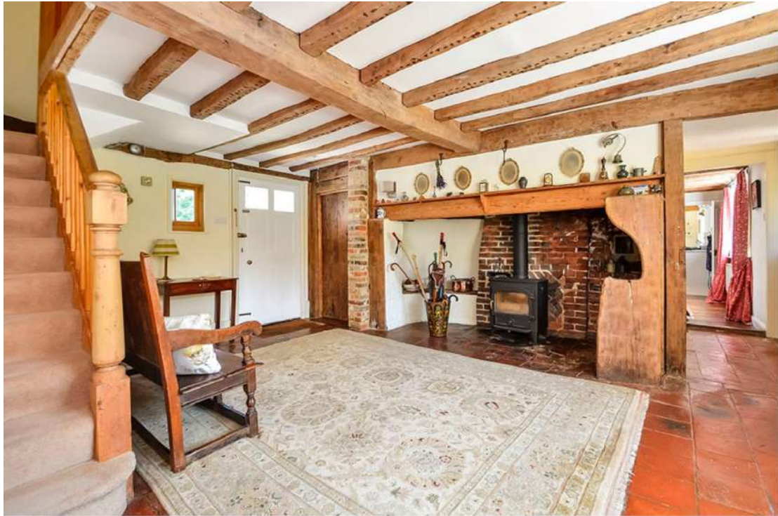
Figure 13; View of the Westernmost of the ground floor rooms in the original core of the house, showing the smoke bay and the later first floor. The modern softwood staircase is visible on the left. Image by Knight Frank.
