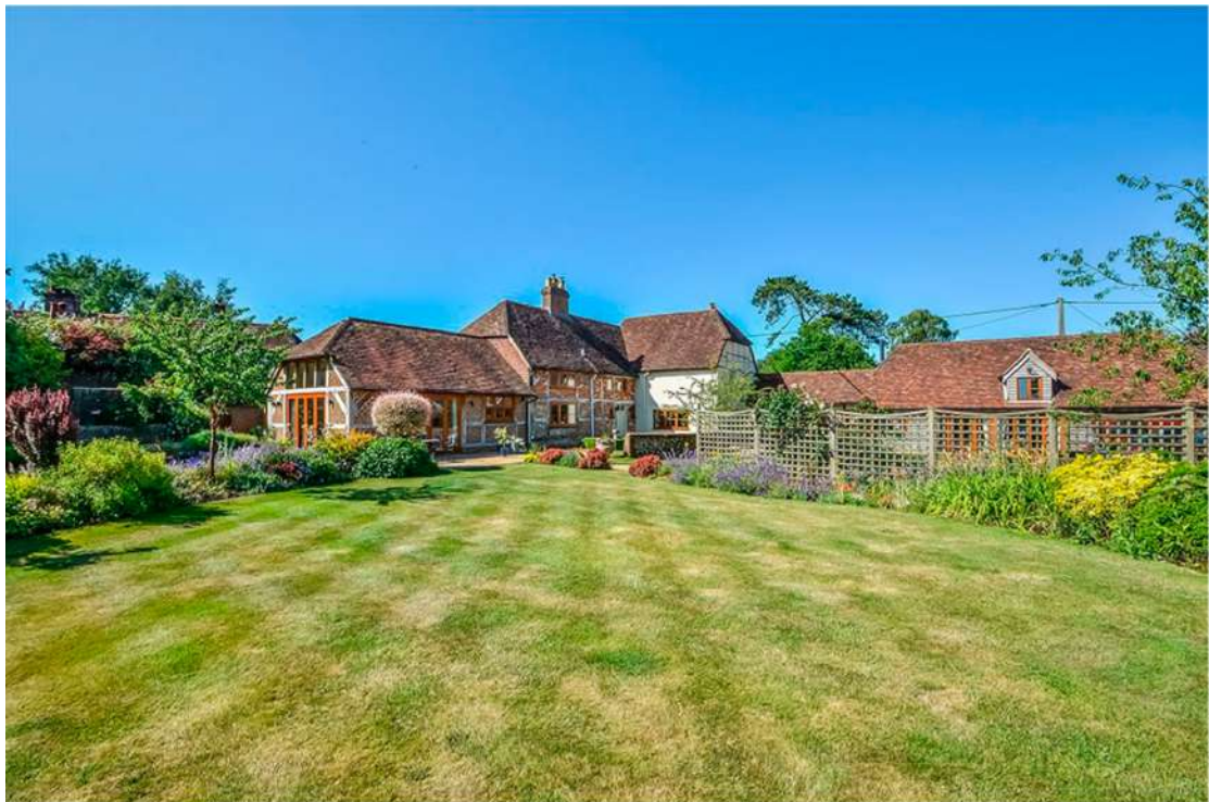
Figure 8; View of the rear (North) elevation of the Farmhouse and the Eastern elevation of the former cart shed, as viewed from the garden. Prominently visible in the left foreground is the kitchen extension, consented in 2011. Image by Knight Frank.
