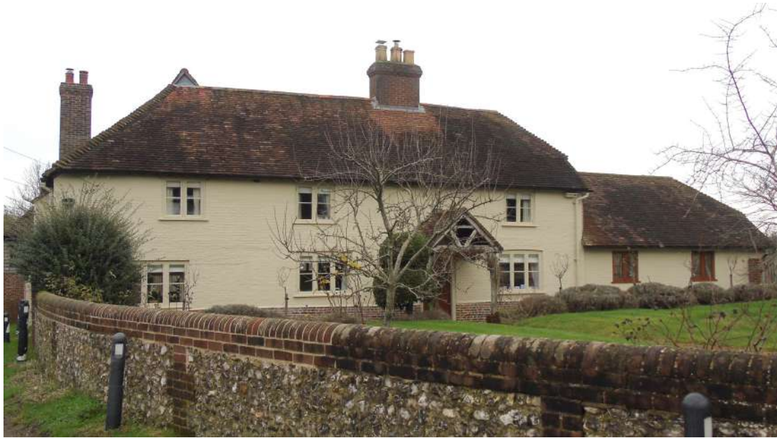
Figure 7; View of the front (South) elevation, as seen from Church Street.
