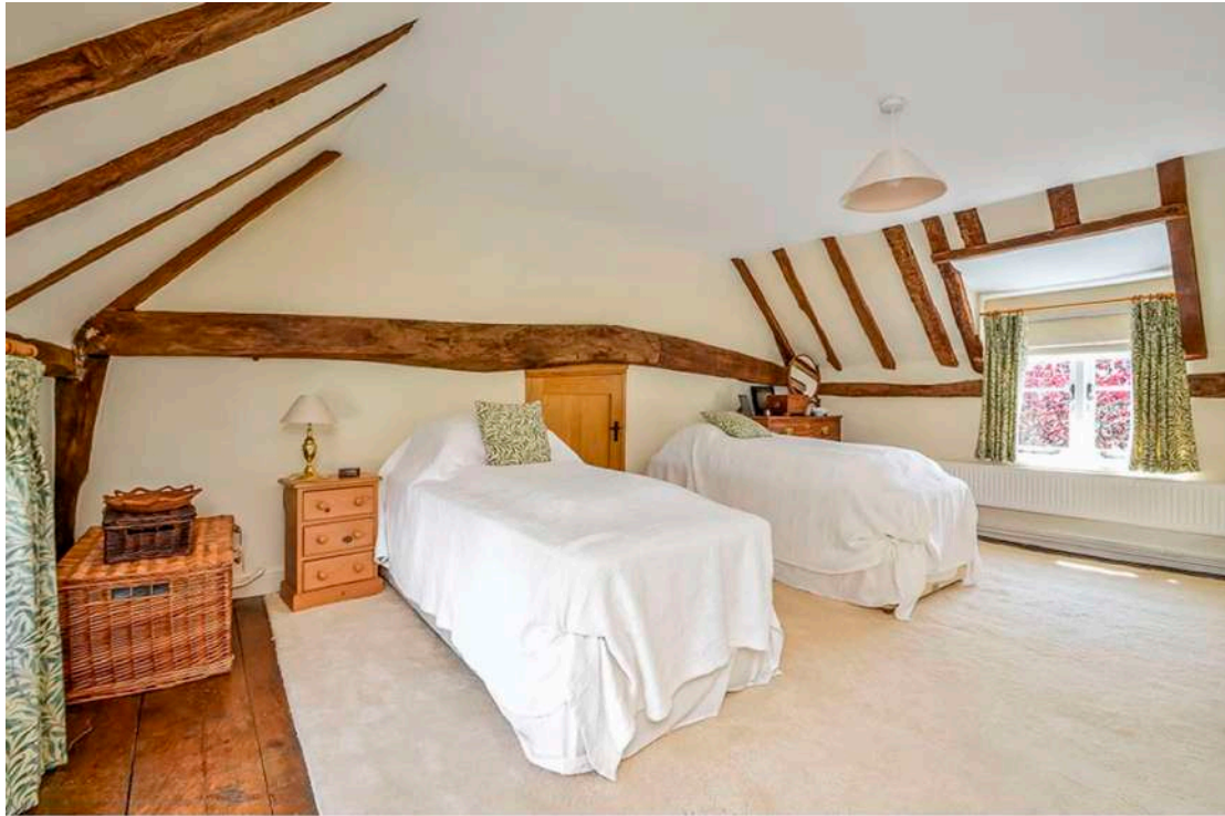
Figure 21; View of the Easternmost bedroom in the historic core of the property. An example of the low accesses and tie beam heights is put into scale by the adjacent beds. Image by Knight Frank.
