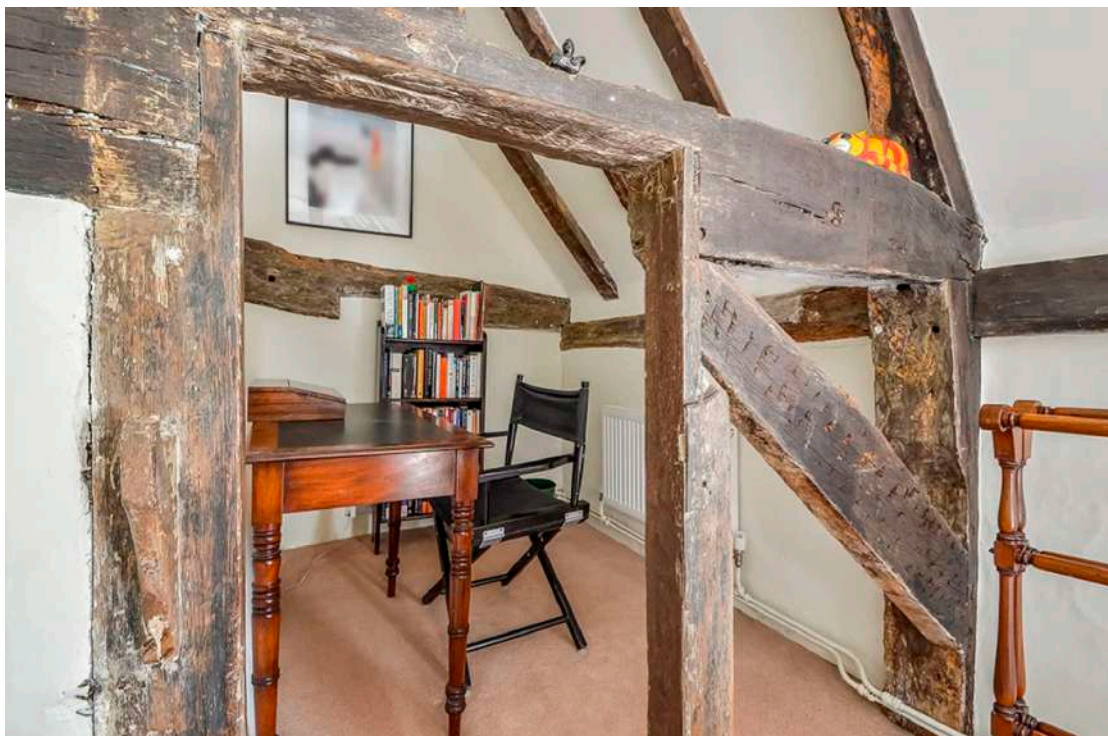
Figure 22; View of the section of the Western bedroom in the historic core of the property, showing the section 'cut-off' between two tie beams and the chimney stack. The furniture illustrates the very low heights of the beams. Image by Knight Frank.
