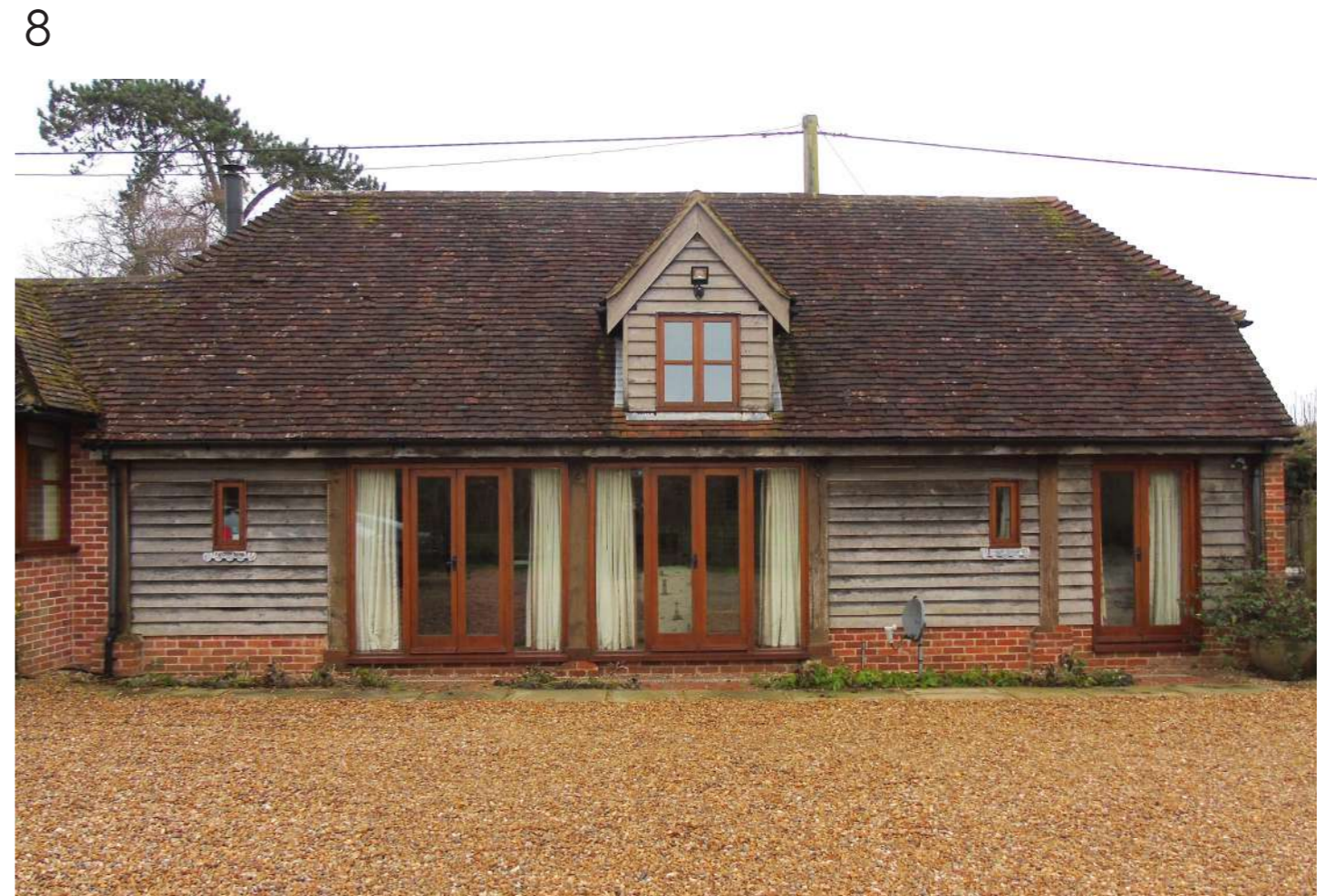
View of the West elevation of the converted former cart shed, as seen from the current drive.
