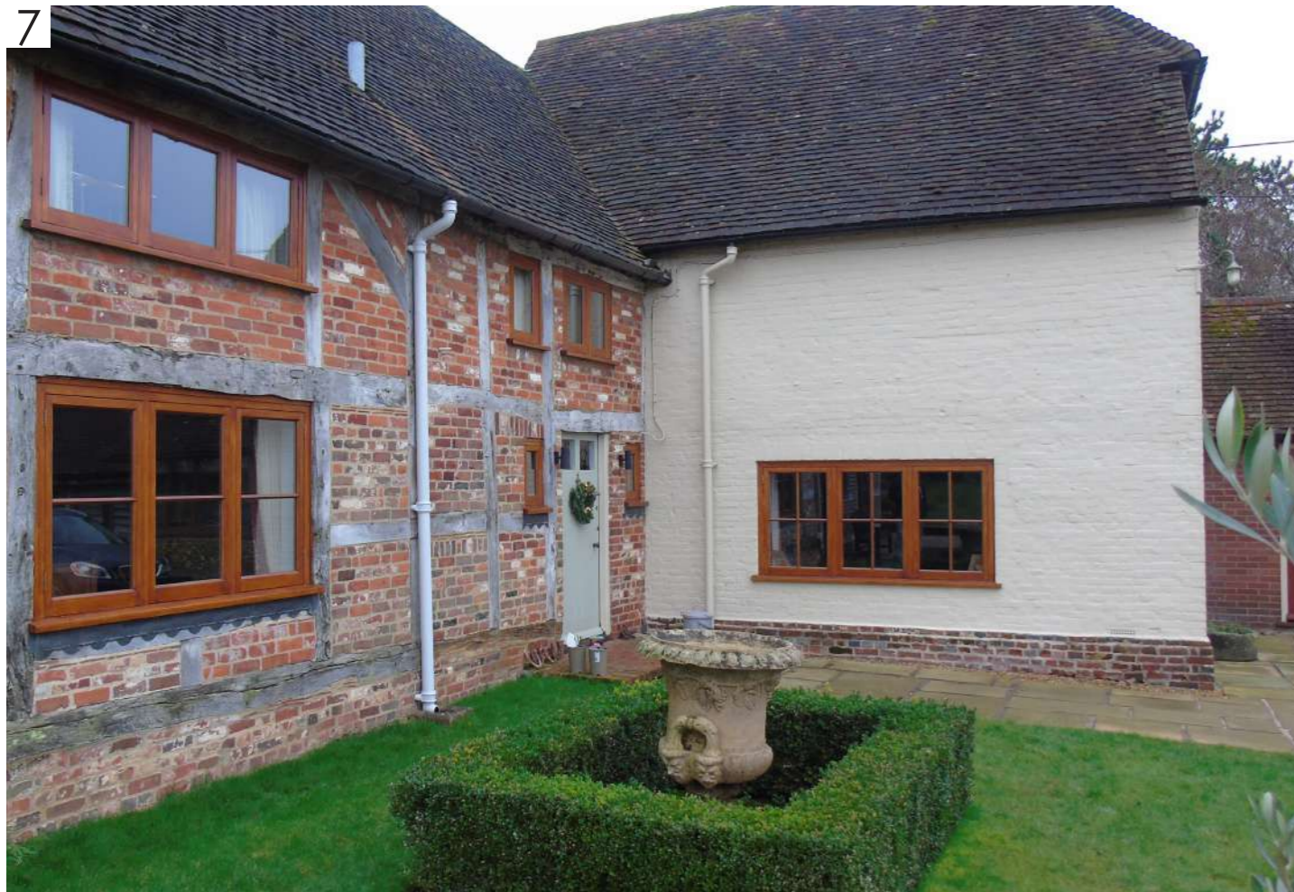
View from the garden of Town Street Farmhouse, looking toward the Eastern elevation of the C18 wing, with painted brickwork.
