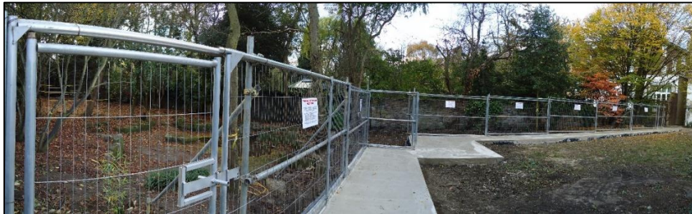
Figure 5. Photograph to illustrate installed protective fencing.
