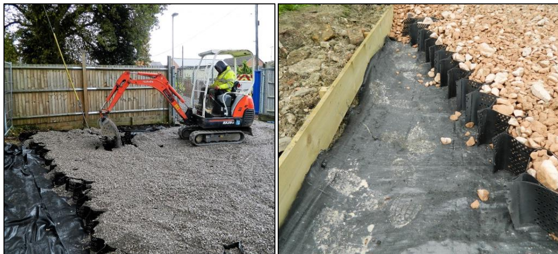
Figure 8. Photographs illustrating cellular confinement system used to form an above-ground no-dig driveway.
