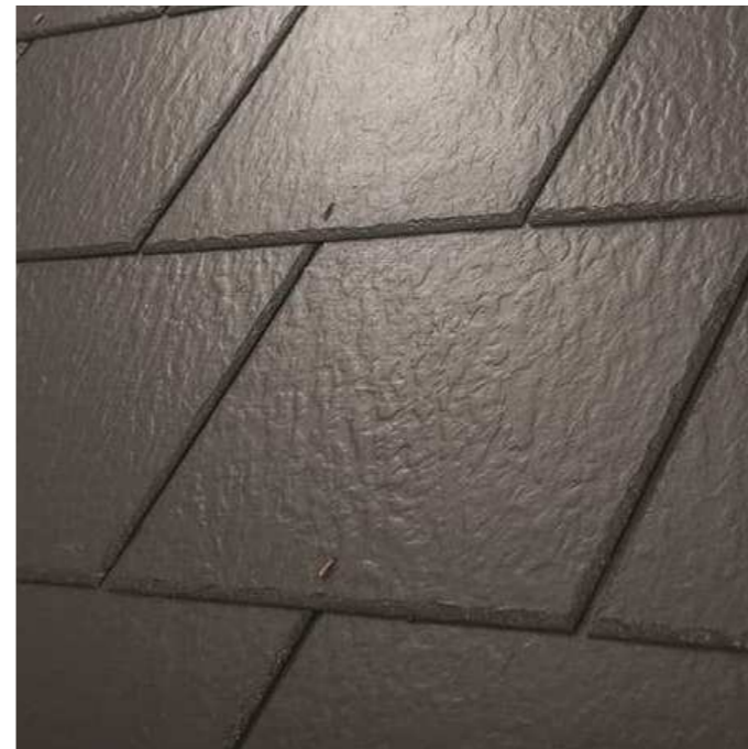
Composite riven slate tiling
