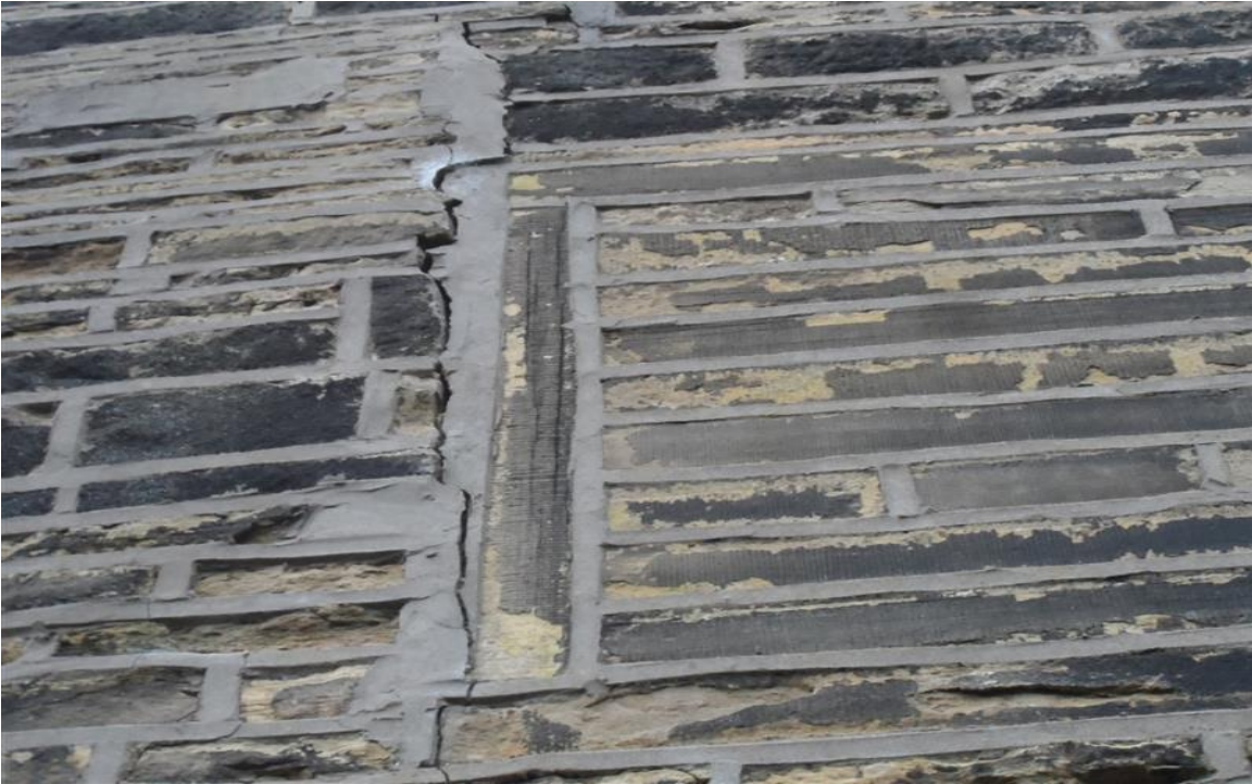
Blocked window right gable 2
