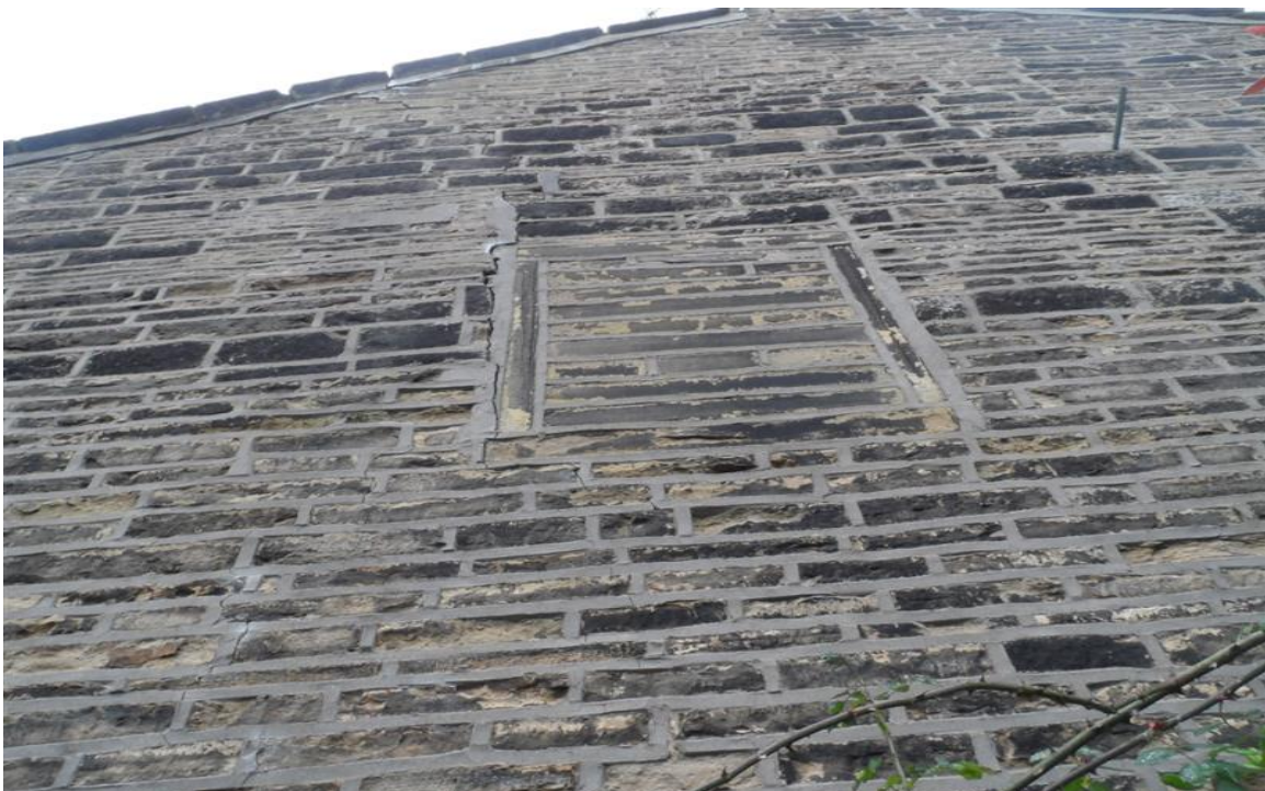
Blocked window right gable 1
