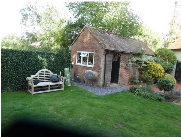
The existing structure.
