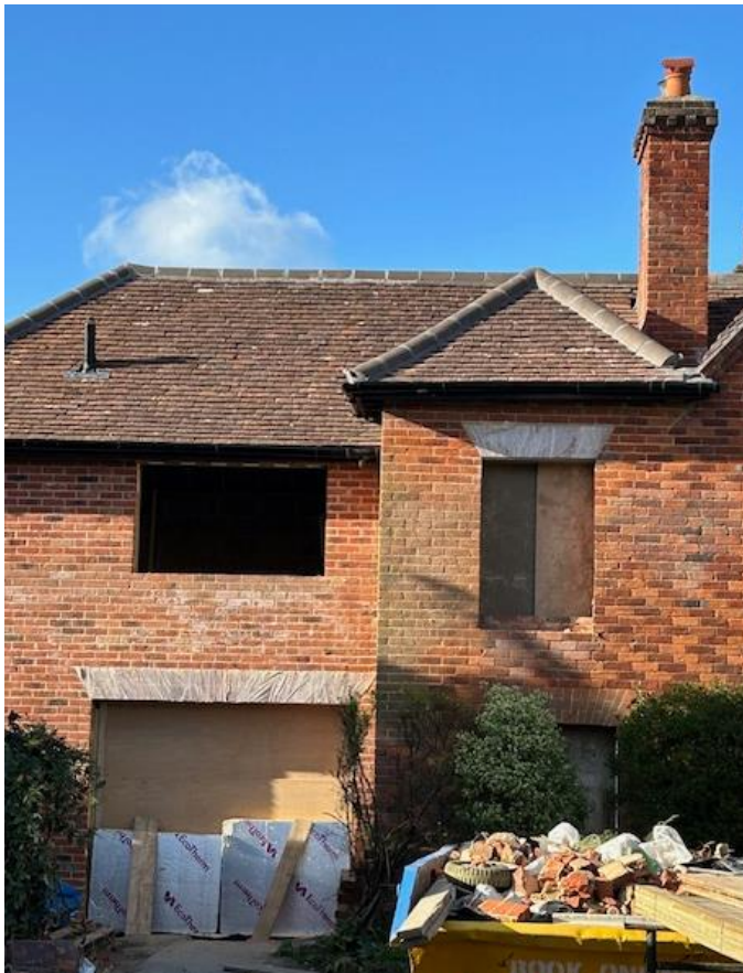
Photos of new roof arrangement
