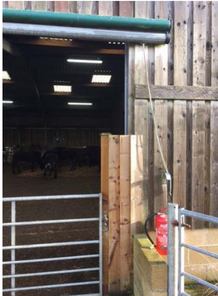
5. Proposed timber cladding style with blockwork base.
