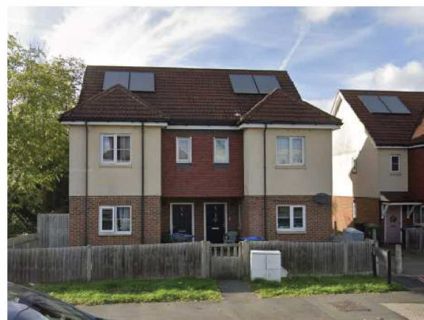
22. Render, Brick and Tile Facade, Kelsey Close neighbouring site
