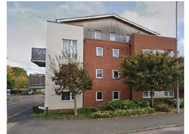
18. Brick, Render and Timber clad facade, Harrow Close, large residential scheme
