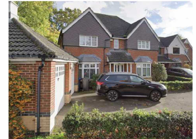
21. Newer developed area, contrasting brick type details, leaded splayed bays, and tiled front full height gables.
