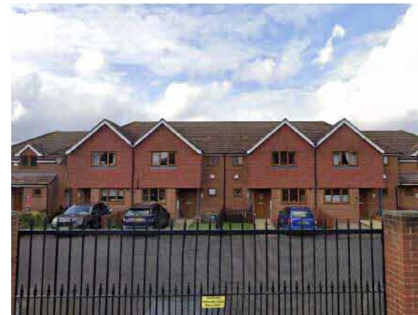
28. Local traditional style terrace housing with tile gable fronts and sheltered entrances.
