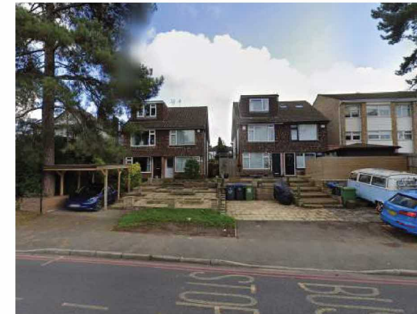
20. Detached tiled and brick front houses with dormers in roof.
