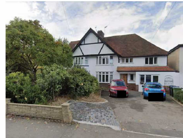
17. Intersecting steep pitched mock tudor gable roof to hip roof, with a half timbering front, leaded glass works.
