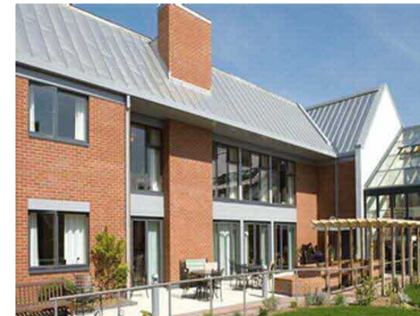
29. Local residential home, Chessington. Zinc roof with modern formed bay fronts.
