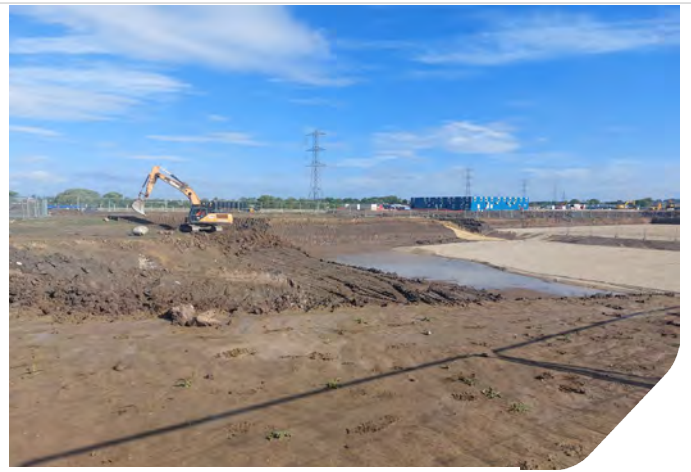
Photo 02: Attenuation basin being trimmed
