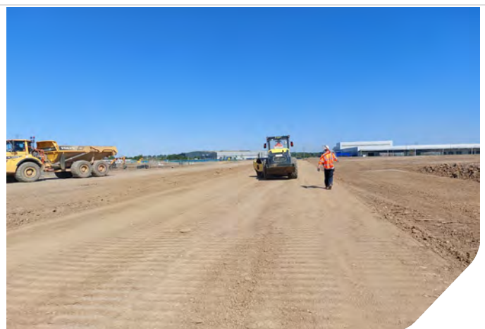
Photo 06: Exploration testing engineer pacing out 50m for CBR test placement
