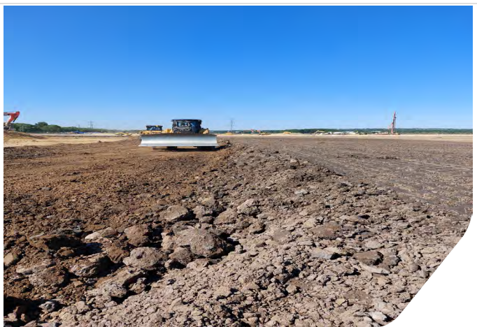
Photo 14: Bulldozer distributing material within Zone 8
