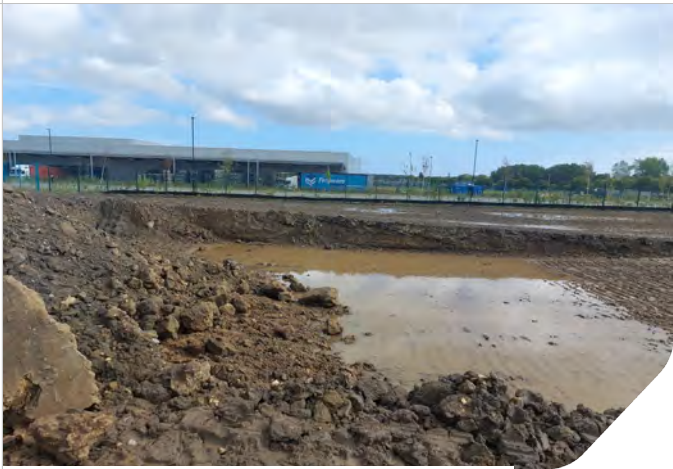
Photo 03: Standing water within dock leveller in Zone 8
