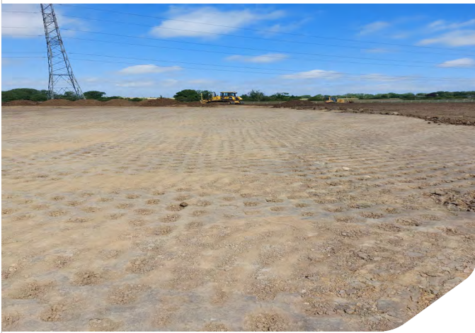
Photo 01: padfoot rolled surface of northwest cell in Zone 3
