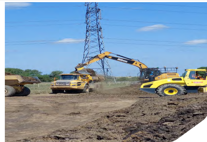
Photo 06: Removal of topsoil bund from the west of cell 6
