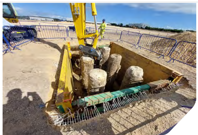
Photo 12: Piling trench in Zone 2
