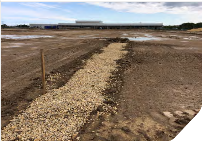
Photo 05: Drainage being placed beneath the piling mat in Zone 5.
