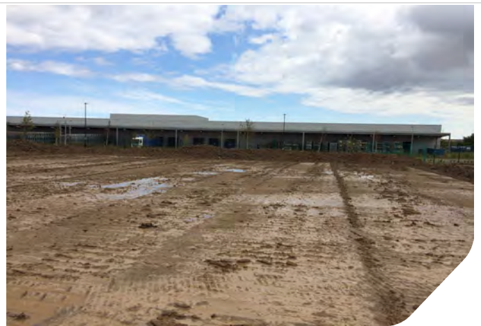
Photo 06: Wet surface area in zone 7 & 8
