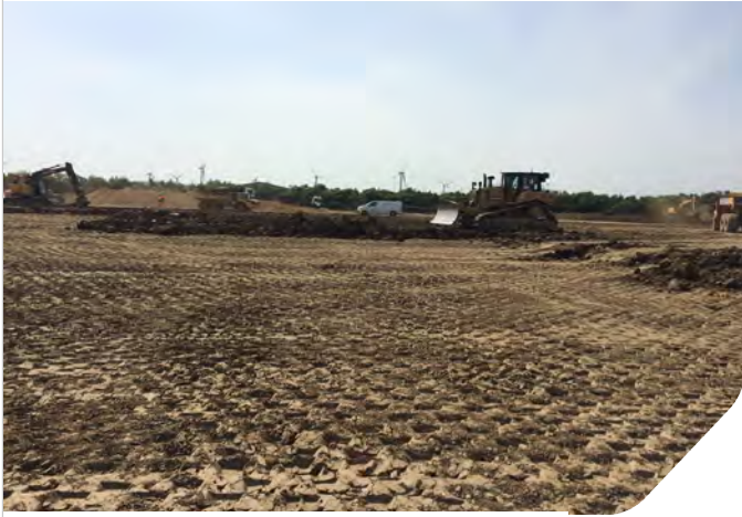
Photo 01: General look across zone 7, showing placement of layer 2.
