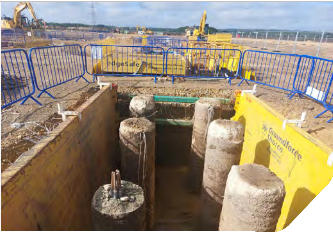
Photo 03: piling cap within Zone 2
