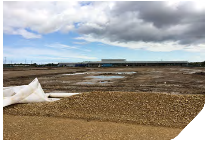
Photo 04: Piling mat placement on edge of Zone 5.
