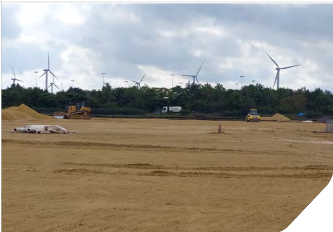
Photo 05: Zone 5 piling mat
