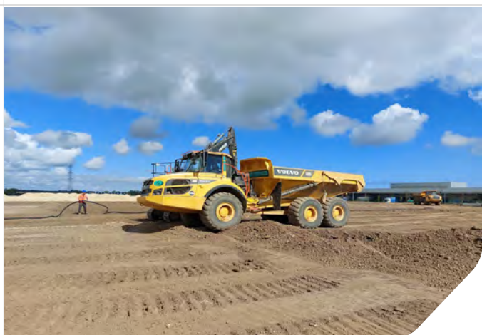
Photo 11: Drainage channel infilling
