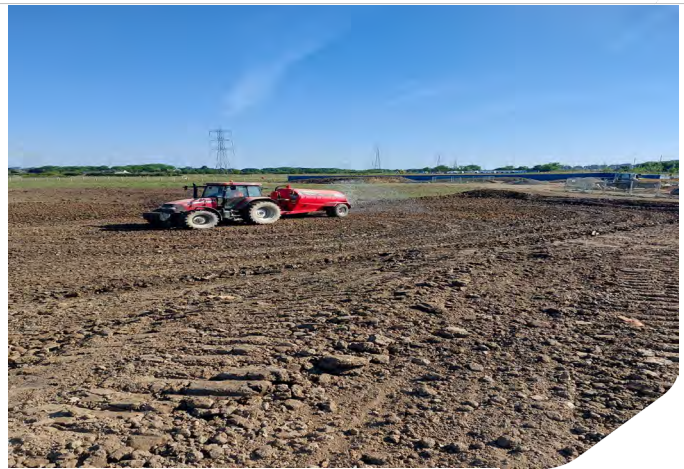
Photo 04: Tractor distributing water over cells 2 and 3
