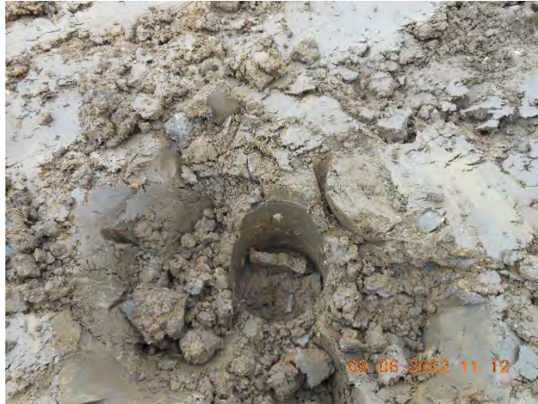
Figure 9. Void left in compacted material following removal of core cylinder.
