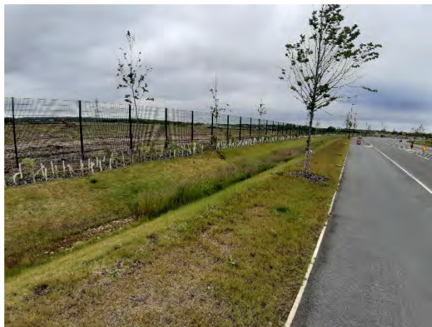
Figure 10. Longitudinal view along eastern boundary along Internation Drive.
