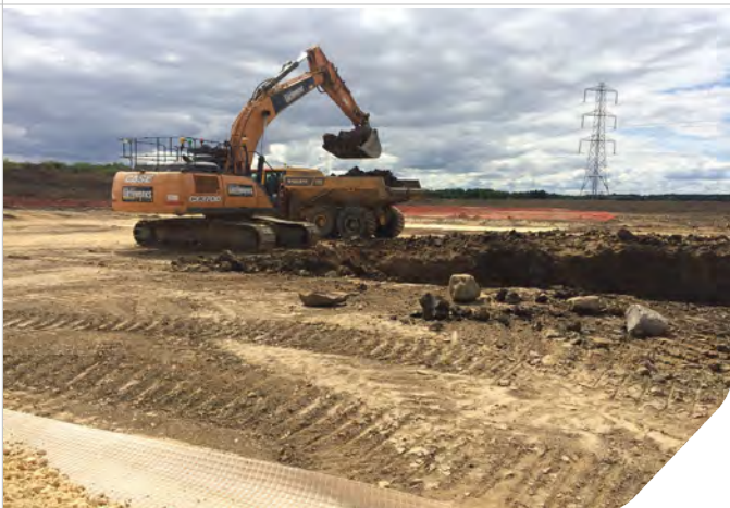
Photo 11: Excavation of cut material in Zone 6, where Cut is deeper due to dock loaders.
