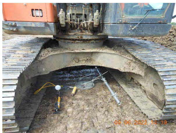
Figure 20. Plate Bearing Test using tracked excavator as kentledge.
