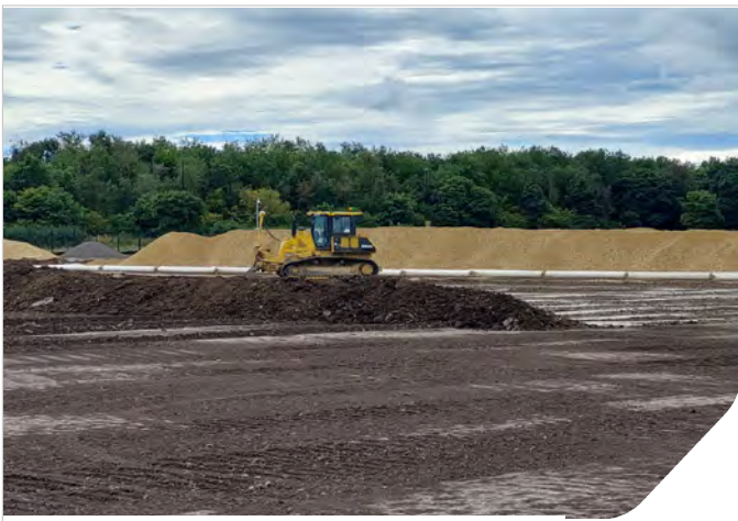
Photo 07: Bulldozer trimming final layer within Zone 8
