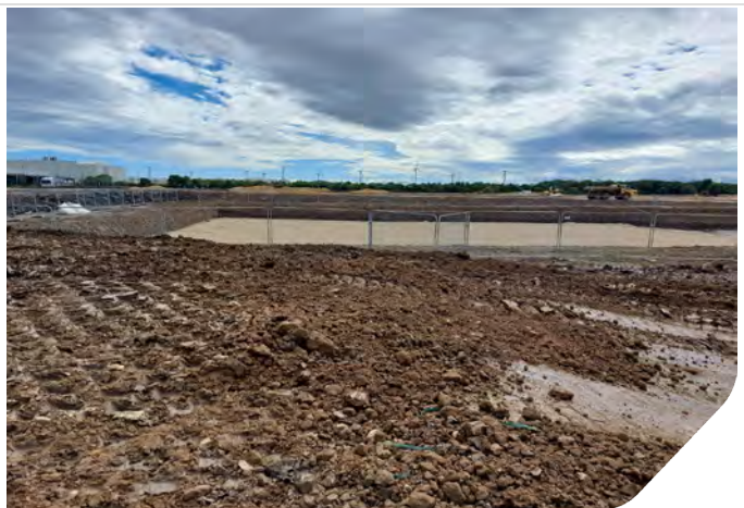
Photo 06: View of attenuation basin facing south
