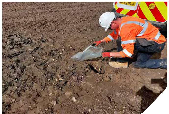
Photo 06: Core cutting testing in Zone 9
