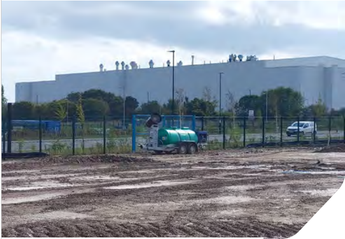
Photo 07: Mist canon on site perimeter
