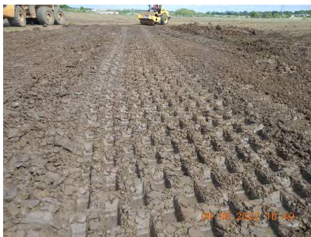
Figure 3. Vibration compaction of first layer of excavated material with Padfoot roller.
