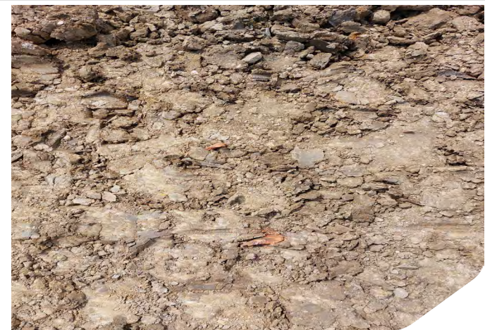
Photo 12: Padfoot rolled surface of cell 3 with evidence of land drains
