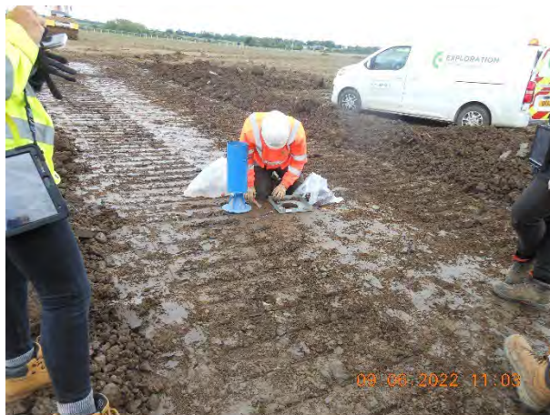
Figure 5. Removal of material for Sand Replacement test.
