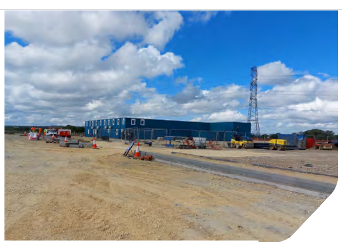
Photo 02: Wates new offices under construction
