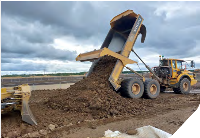
Photo 03: Dump truck delivering excavated material from Zone 4 to Zone 6
