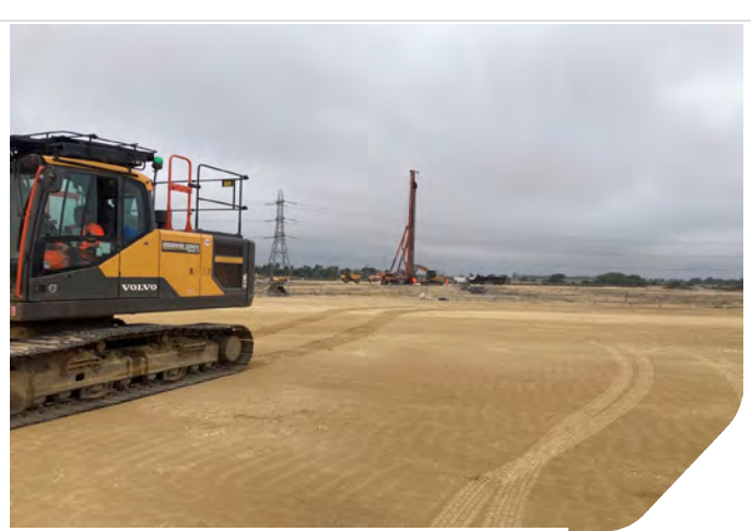
Photo 02: CBR test in relation to current location of piling rig
