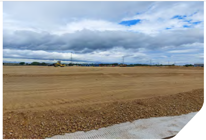
Photo 10: Compaction of piling mat in Zone 7
