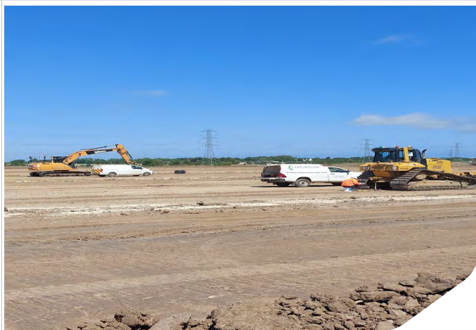
Photo 05: Exploration technicians undertaking plate load testing in Zone 2
