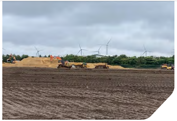
Photo 10: Bull dozer distributing conditioned clay in Zone 8
