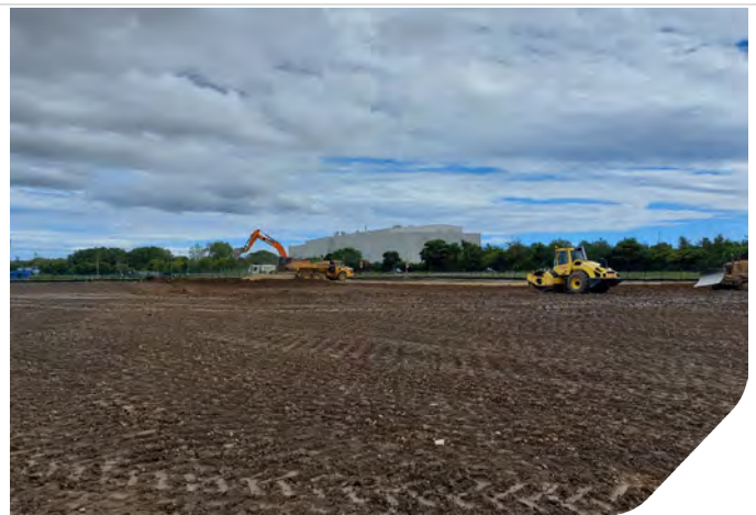
Photo 12: View of type 1 stockpile being transported and padfoot rolling of Zone 8
