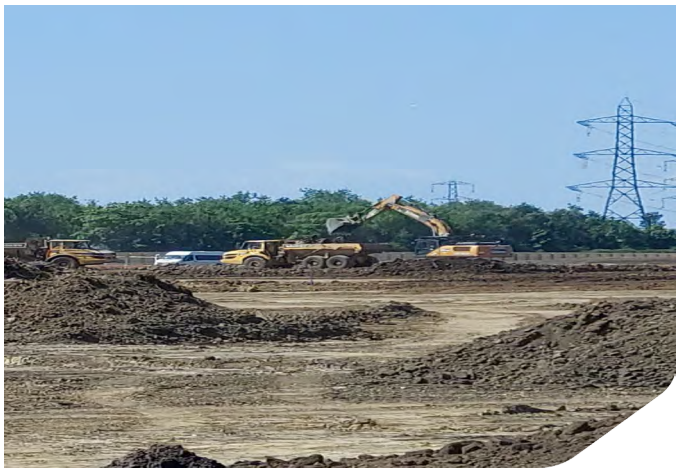
Photo 02: Cut from Zone 2 being transported to Zone 3
