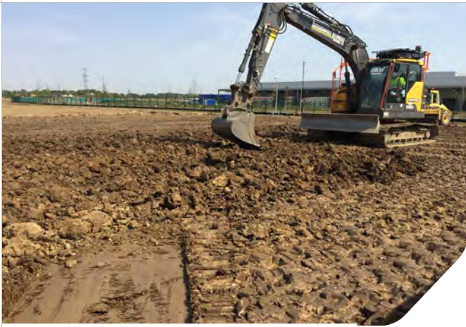
Photo 03: excavator mixing the placed materials to add moisture prior to rolling.
