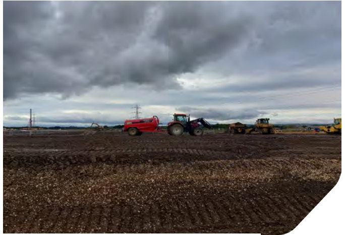
Photo 02: Tractor with bowser distributing water in Zone 6
