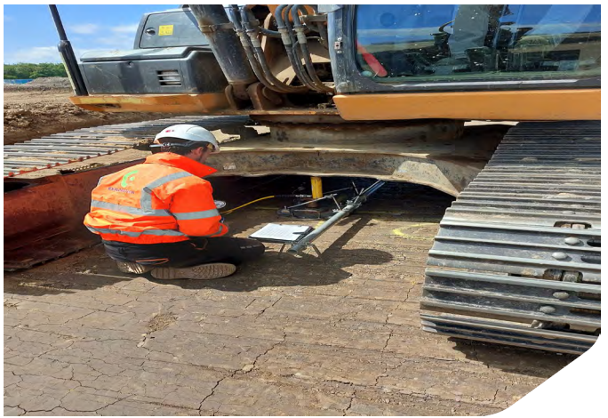
Photo 02: Plate load test in Zone 2
