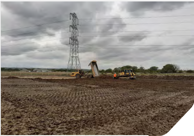
Photo 01: Placement of fill material in Zone 3
