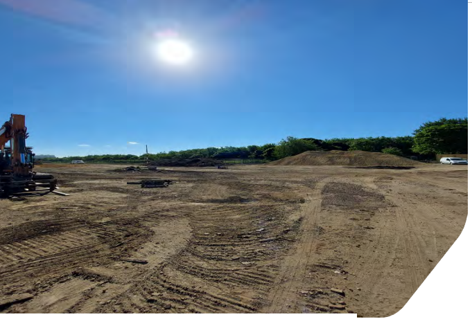
Photo 09: Smaller stockpile for temporary road surface
