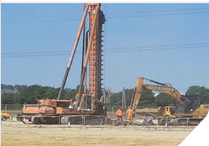
Photo 11: Piling rig in Zone 2
