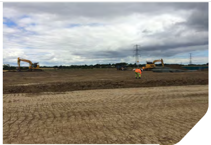
Photo 02: Placement of fill (layer 1) in Zone 7.
