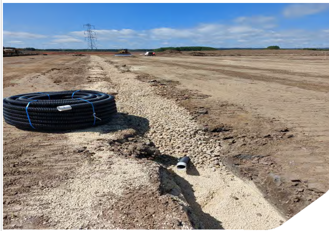
Photo 11: End of the drainage pipe within Zone 2
