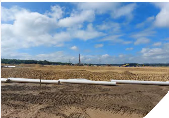
Photo 05: Edge of piling mat within Zone 5
