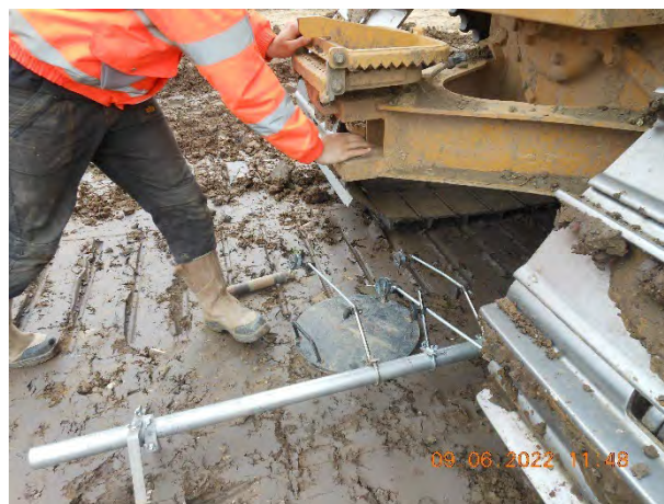
Figure 13. Plate Bearing Test being set up below dozer.
