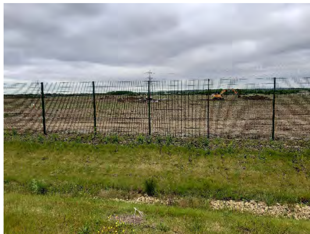
Figure 7. Topsoil strip area inside of site boundary adjacent to International Drive.
