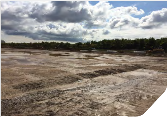
Photo 01: General view across Zone 5, showing finished cut level and pooled standing water from heavy rains.
