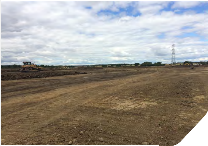
Photo 15: General view across Zone 7 from Zone 3.
