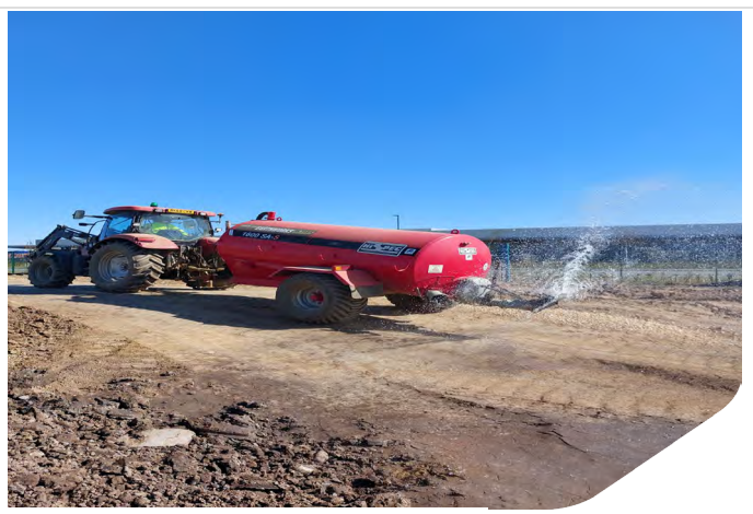
Photo 12: Tractor undertaking dust suppression on roadways
