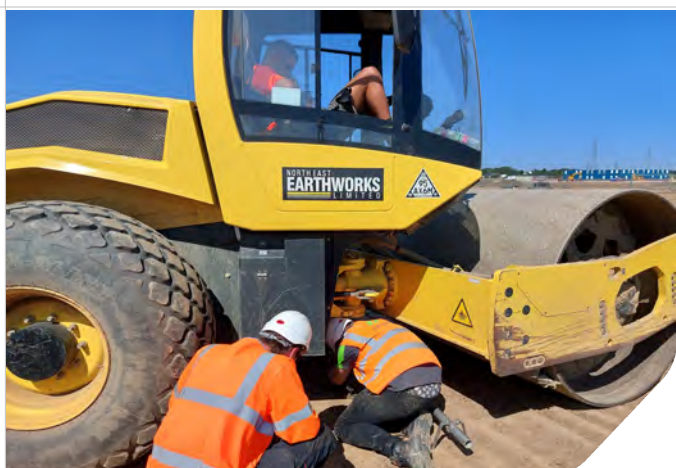
Photo 05: Exploration testing engineers undertaking CBR testing in Zone 6
