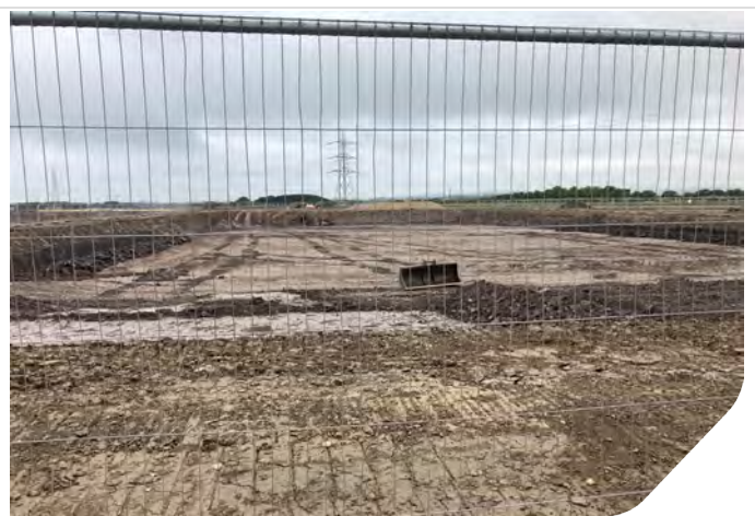
Photo 12: Attenuation basin in Zone 4
