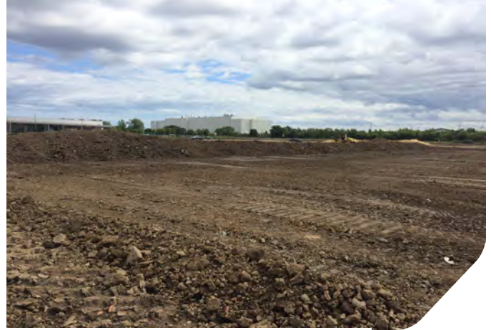
Photo 08: Looking across zone 7 layer 2, the mound marks the edge of the placed fill and the approximate boundary between zone 2 and zone 7.
