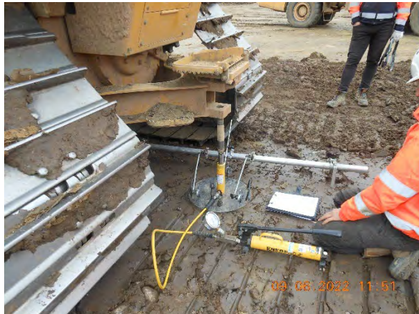
Figure 14. Plate Bearing Test being carried out following fourth pass of layer 1.
