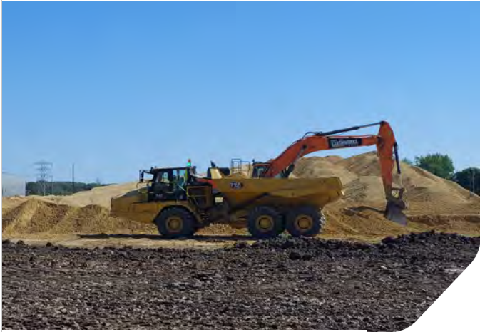
Photo 07: Dumptruck collecting Type 1 from stockpile in Zone 8 and 9
