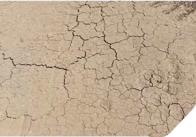
Photo 17: Strata of roadways before dust suppression
