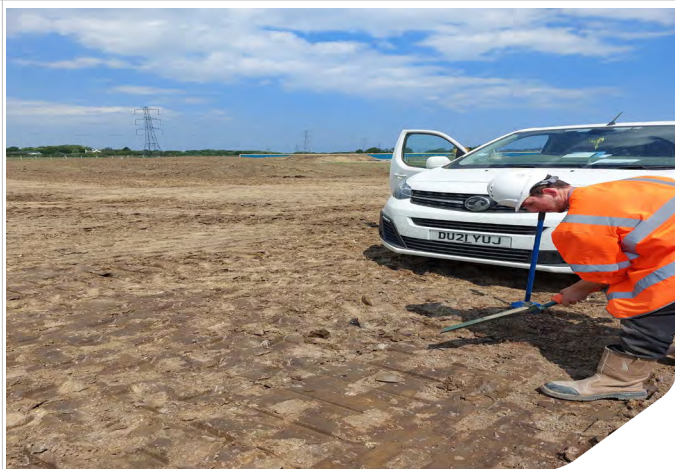
Photo 11: Digging out a core cutter test from location 5
