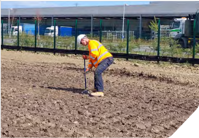
Photo 03: Core cutting testing in Zone 9
