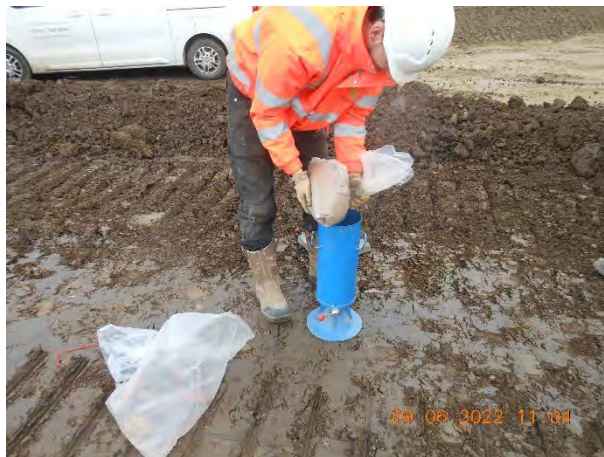
Figure 6. Filling test cylinder with sand.
