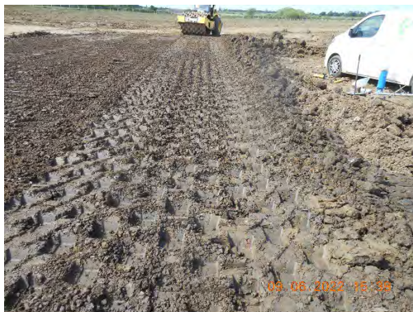
Figure 28. Layer two compaction during passes one and two.
