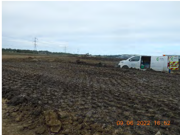
Figure 32. Compacted material following passes seven and eight of layer two.
