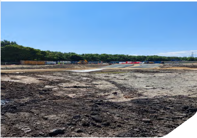
Photo 07: Tarmacked vehicle entrance to site
