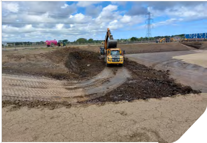
Photo 09: Attenuation basin excavation
