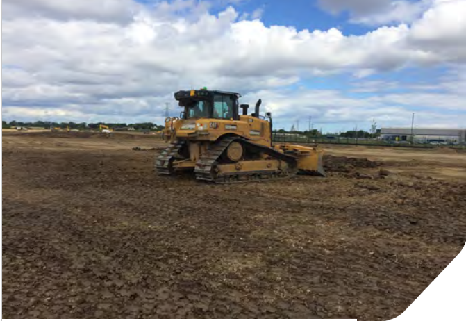
Photo 07: Dozer spreading fill zone 7, layer 1.
