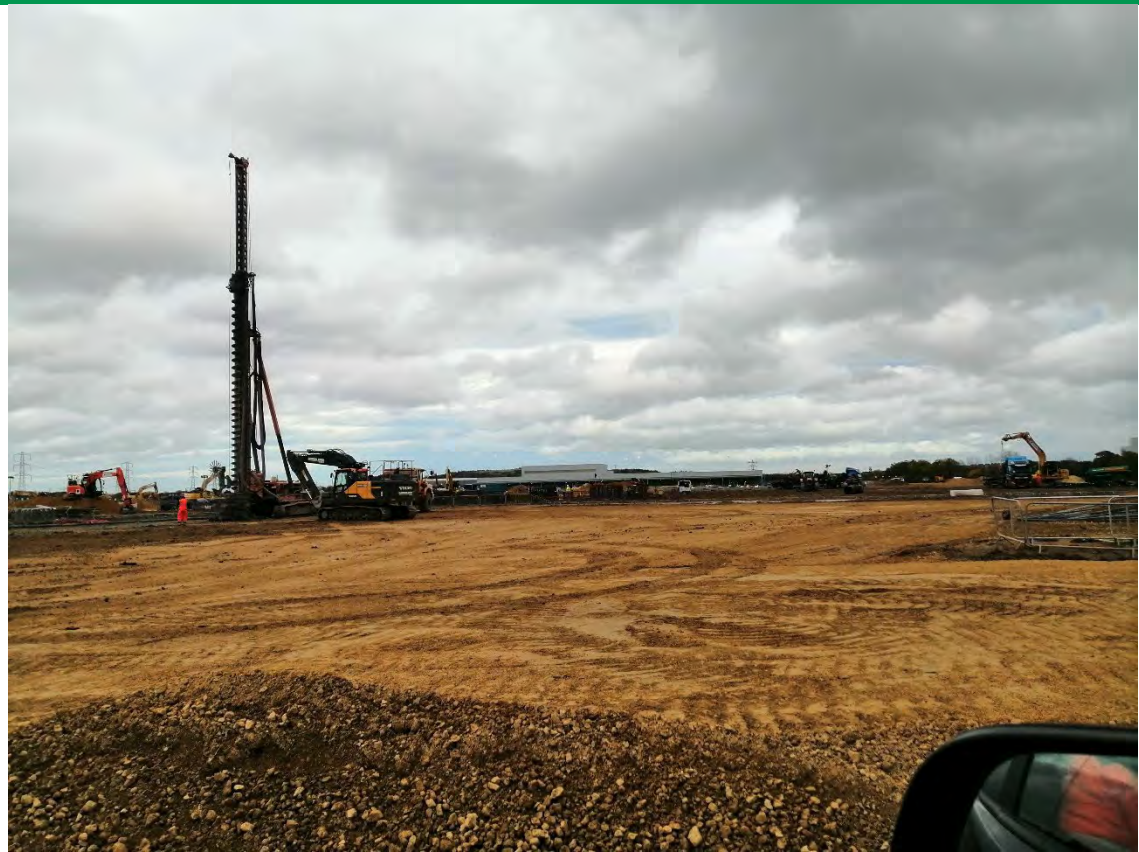
PLATE 2 – PILING WORKS AND CUT SURFACE
