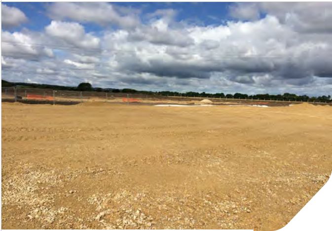
Photo 03: Piling mat in Zone 2.
