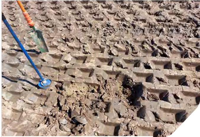
Photo 01: Exploration testing engineer undertaking core cutter tests in Zone 8
