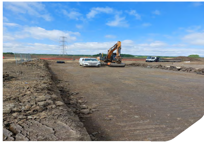
Photo 12: Start of testing within Zone 2 in south west corner
