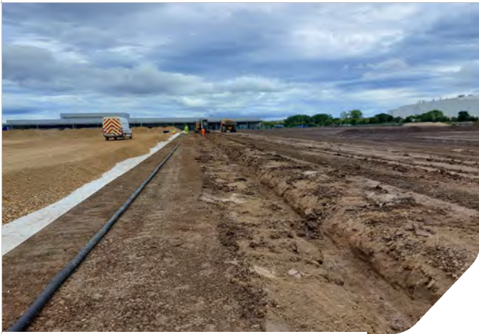
Photo 09: Drainage channels being excavated within Zone 8
