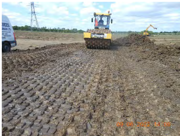
Figure 15. Vibration compaction pass six.
