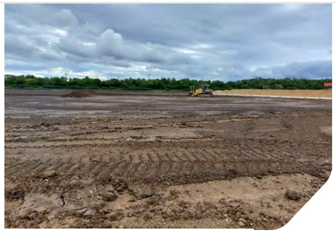
Photo 08: Bulldozer trimming final layer within Zone 8
