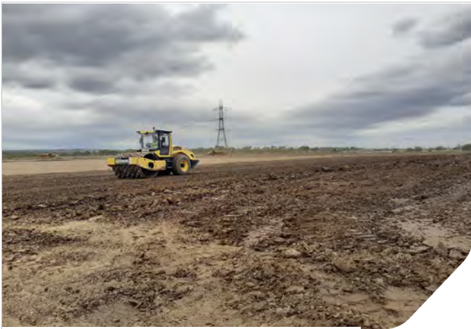
Photo 07: Bomag padfoot roller in Zone 2
