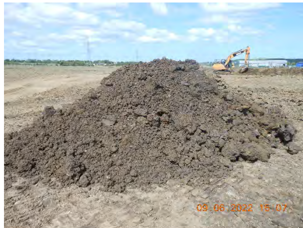
Figure 25. Dumped material for second test layer.
