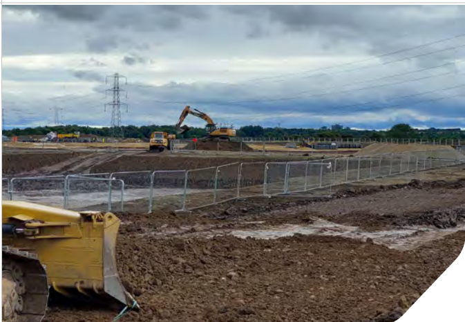
Photo 05: Material being excavated in Zone 4
