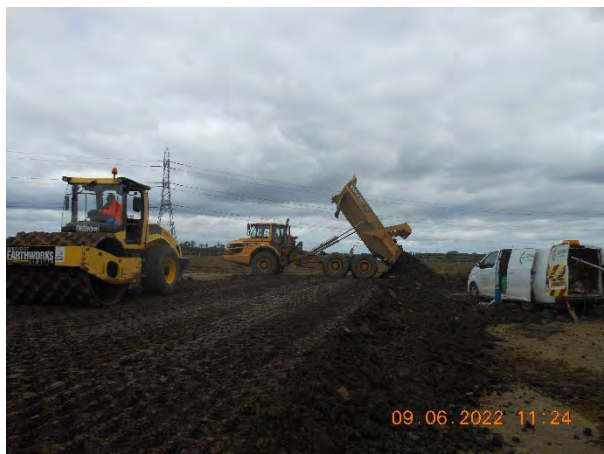
Figure 11. Material being dumped ready for next layer to be levelled out.
