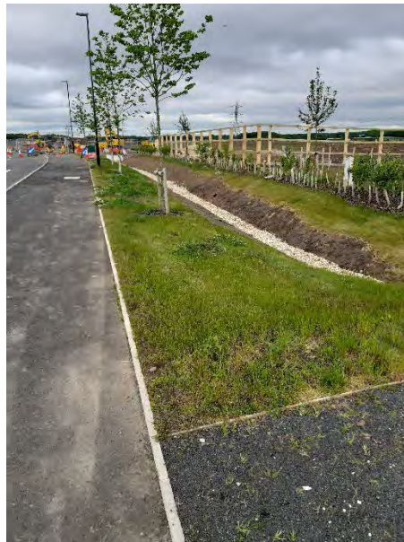
Figure 1. Completed swale running adjacent to public foot path.
