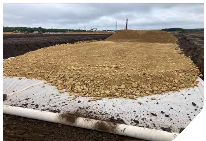
Photo 06: Temporary road surface in Zone 7
