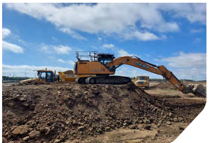
Photo 10: Excavator removing topsoil bund
