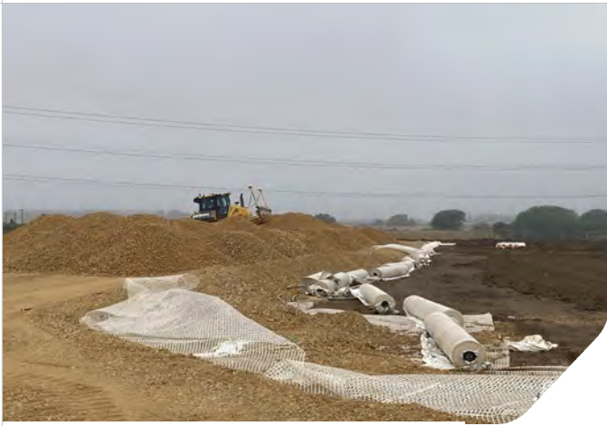
Photo 09: Bull dozer distributing type 1 into Zone 7
