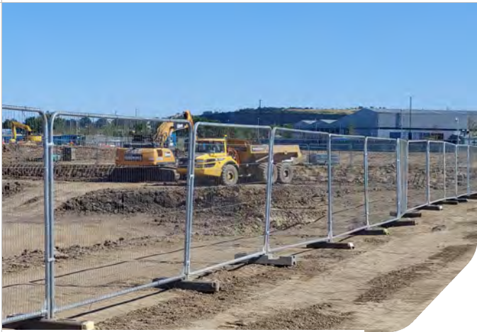
Photo 09: Attenuation basin excavation in Zone 4
