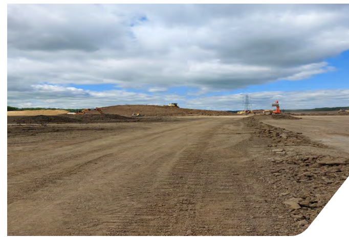
Photo 12: Temporary road leading from stockpile in Zone 7 to Zone 3
