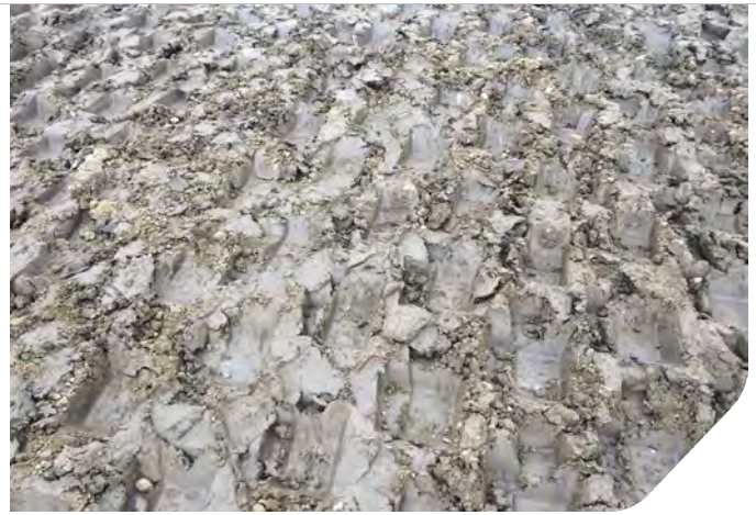
Photo 04: Dimpled surface left by pad foot roller.
