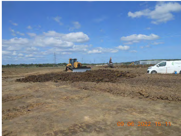
Figure 26. Spreading layer two material.
