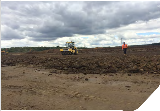
Photo 03: Fill placement in Zone 7, Layer 1.
