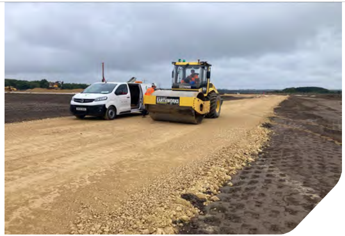
Photo 04: Temporary road surface within Zone 7
