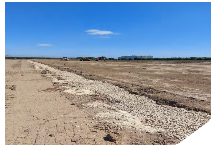
Photo 06: Drainage pipe across Zone 2
