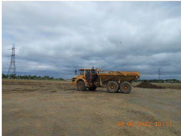
Figure 1. First batch of excavated material dumped at trial area.
