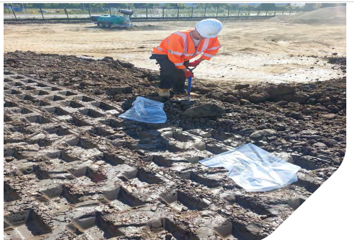
Photo 04: Exploration testing engineer undertaking core cutter tests in Zone 8
