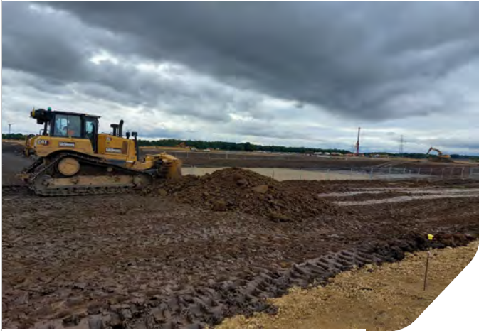
Photo 01: Cat D6 dozer distributing material in Zone 6
