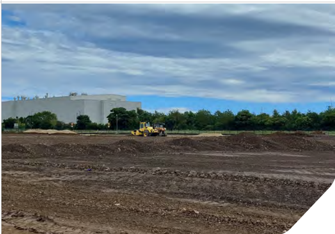
Photo 11: Material in southeast of Zone 8 being rolled
