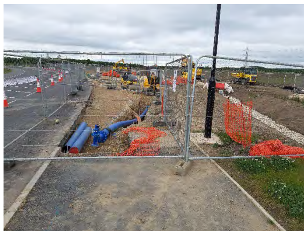
Figure 2. Diversion of existing water main.
