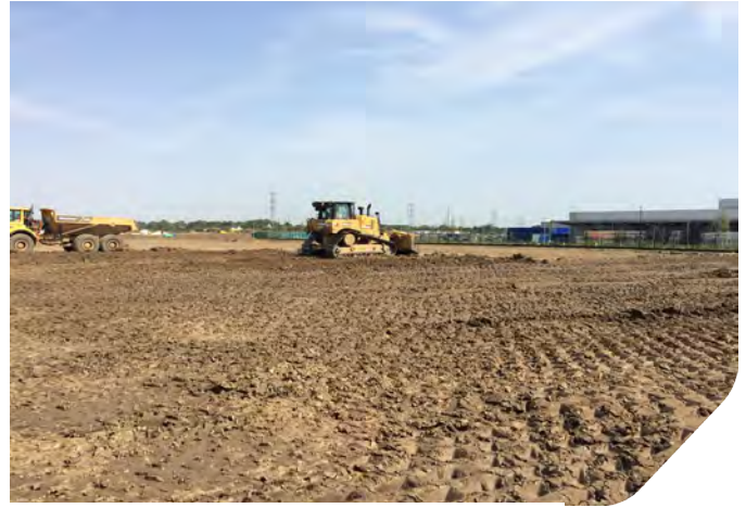
Photo 02: Dozer placing fill in layer 2 in zone 7.
