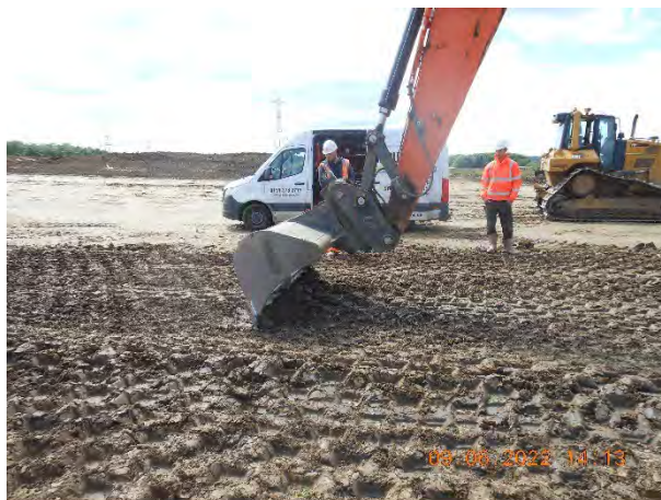
Figure 17. Scraping off dimple material to form flat surface for testing
