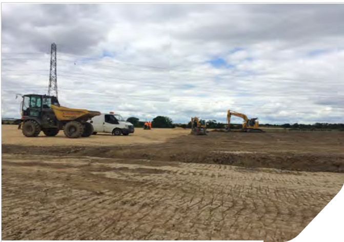
Photo 01: Placement of Type 1 in Zone 3.
