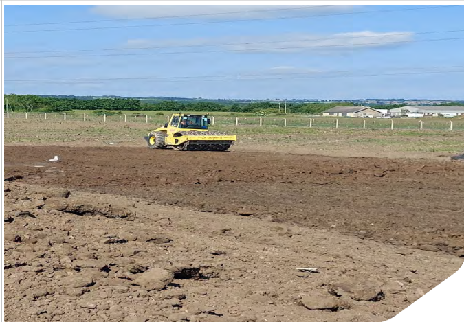
Photo 05: Padfoot rolling of cell 1
