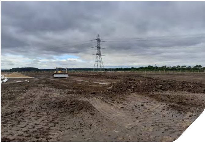
Photo 03: Bulldozer trimming 100mm Zone 6
