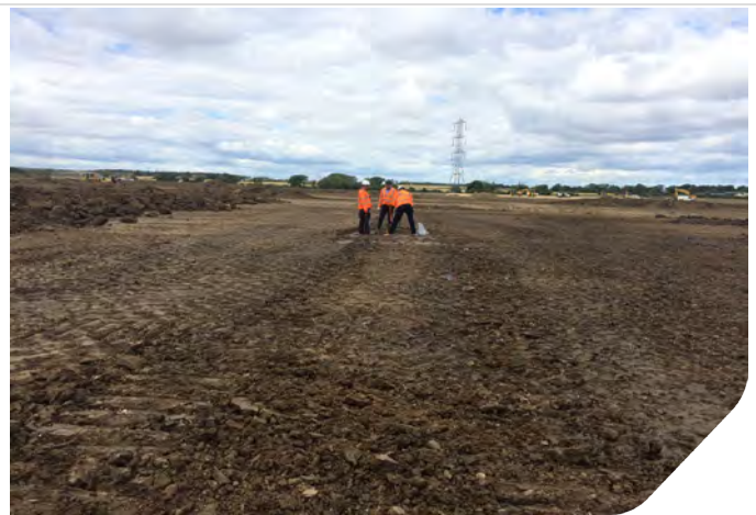
Photo 06: Core cutter test zone 7 layer 1, to the left Layer 2 is visible.
