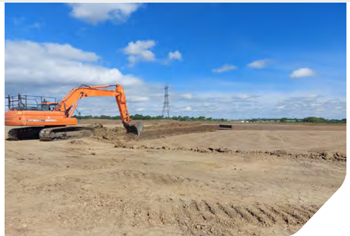
Photo 06: Excavating material from Zone 2
