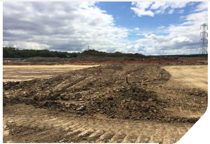
Photo 14: Small stockpile of topsoil to be removed from site.
