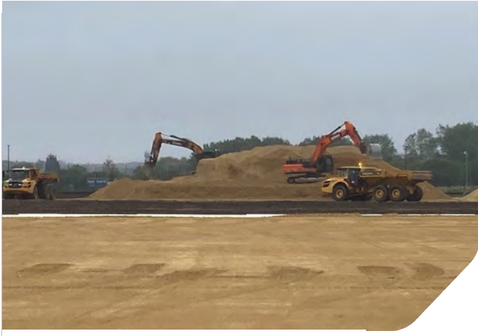
Photo 07: Type 1 stockpile in Zone 8 and 9
