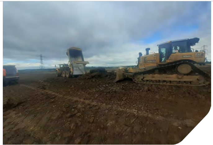
Photo 04: Placing material in Zone 4
