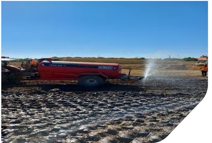
Photo 16: Tractor with water bowser distributing water to Zone 8
