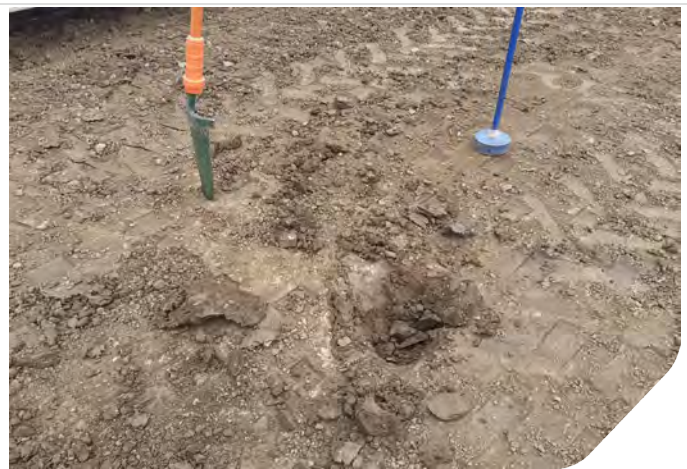
Photo 12: Area of removed Core
