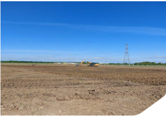
Photo 01: Scarifying of cell 6 in Zone 3
