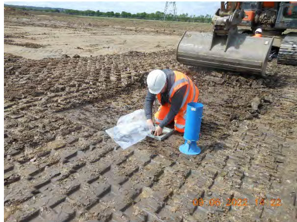
Figure 21. Collecting soil sample for Sand Replacement test.
