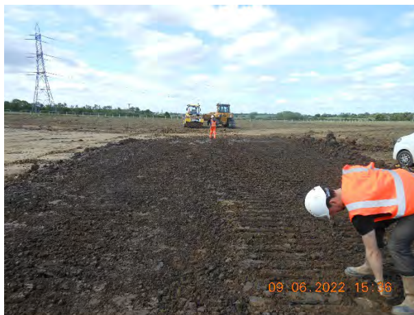
Figure 27. Layer two material levelled prior to compaction.
