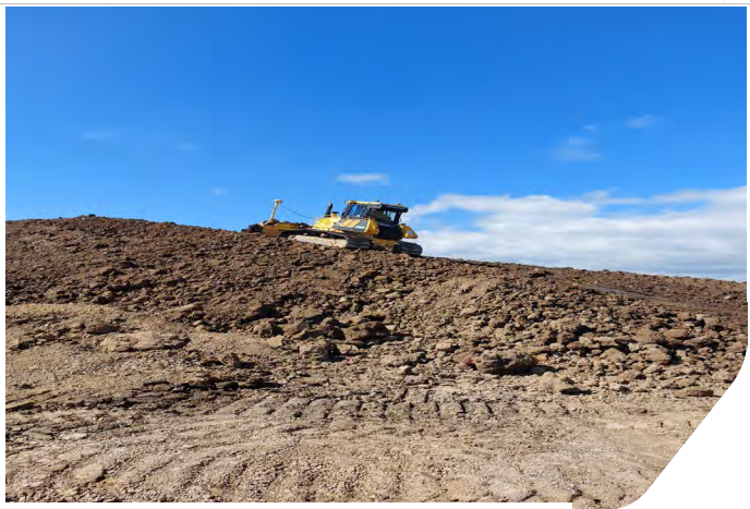
Photo 04: Stockpiling of cut material from Zone 2
