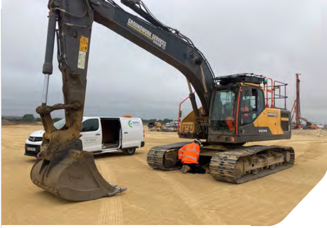
Photo 01: CBR test on piling mat in Zone 5
