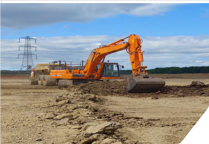
Photo 05: Excavating material from Zone 2
