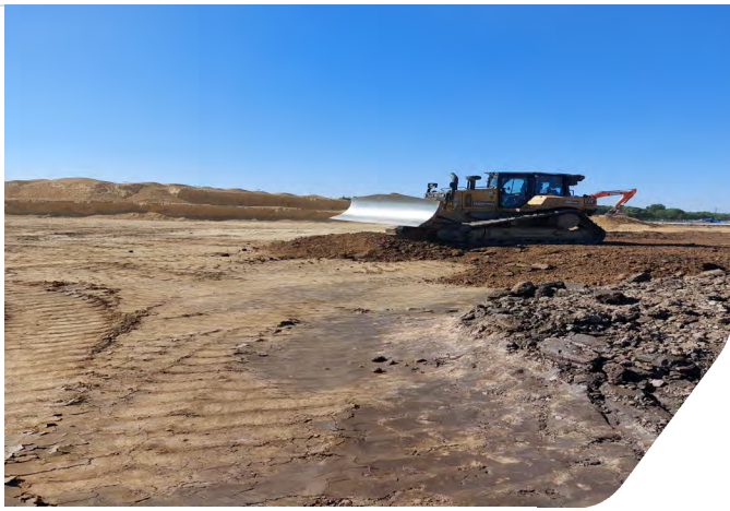
Photo 13: Bulldozer distributing material within Zone 8
