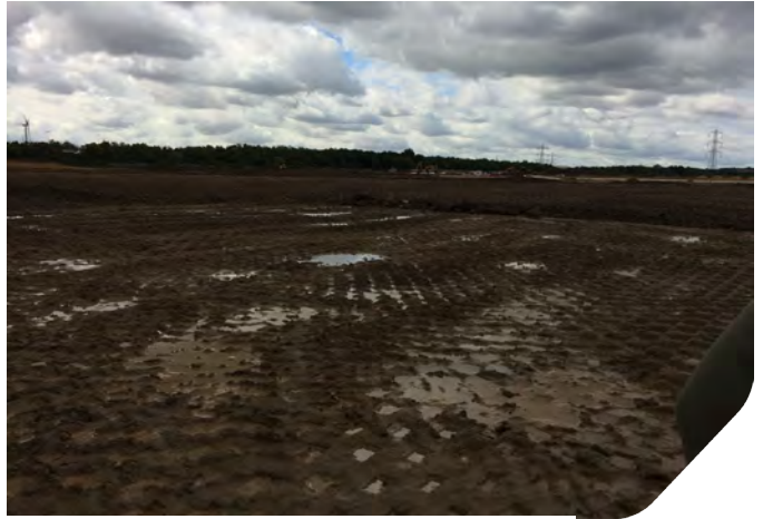
Photo 08: Pooled water in dimples left by padfoot Roller.
