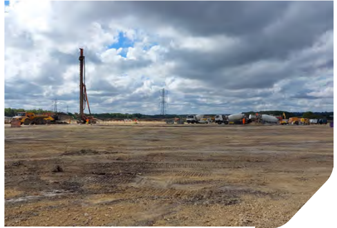
Photo 08: View of piling mat from Zone 10
