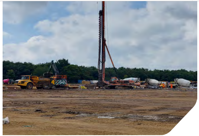
Photo 04: Piling rig in Zone 5
