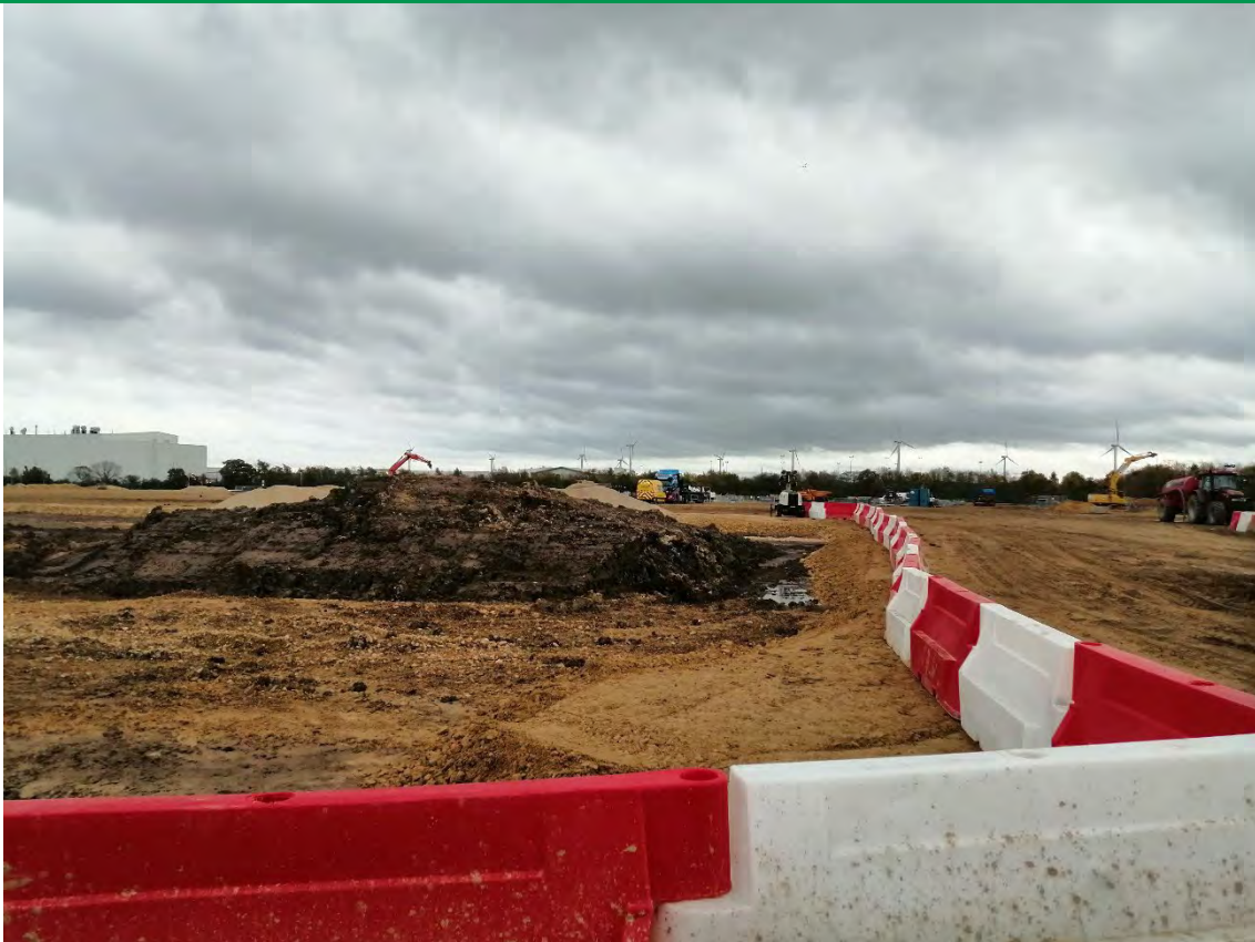
PLATE 6 – COMPLETED LEVELS AND STOCKPILED MATERIALS FOR REPLACEMENT WITHIN CRATE STORAGE SYSTEM IN CENTRAL SITE AREA
