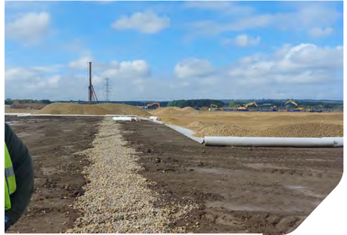
Photo 08: French drainage channels within Zone 8
