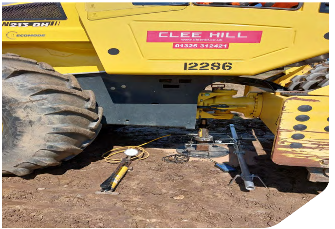
Photo 08: Plate Load Test 1 under Bomag Padfoot roller
