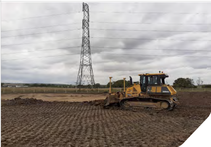
Photo 05: Distribution of fill material
