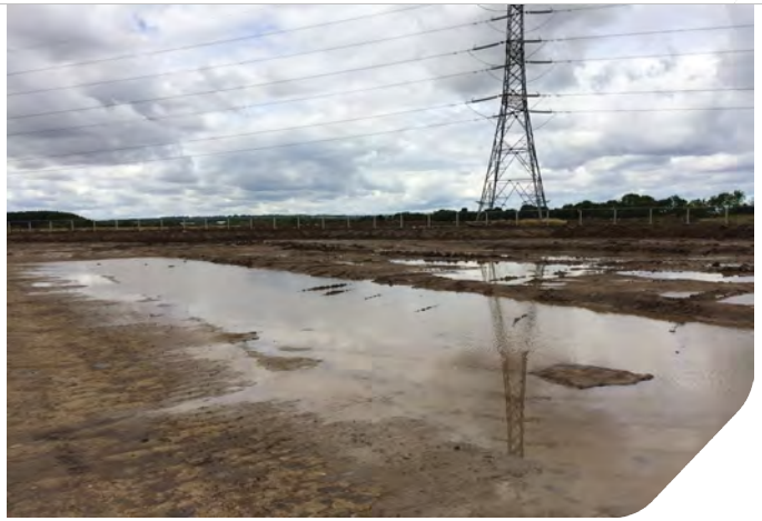
Photo 10: Ponded surface water in zone 6.
