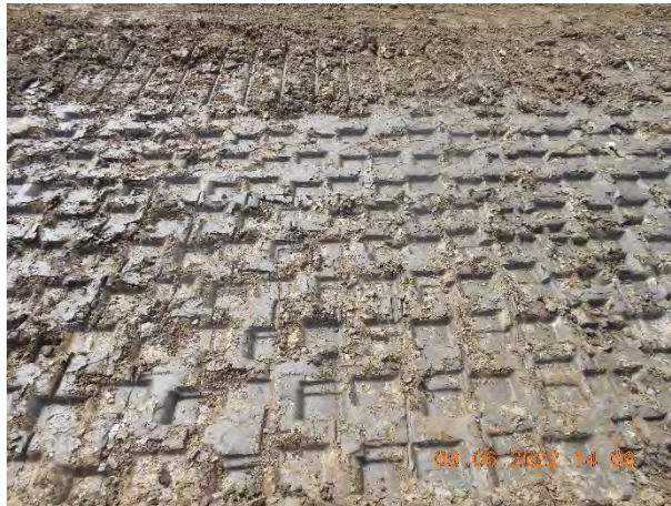
Figure 16. Compacted material following pass six.
