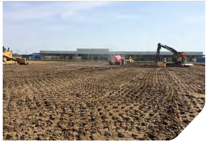
Photo 04: Water added to placed fill.
