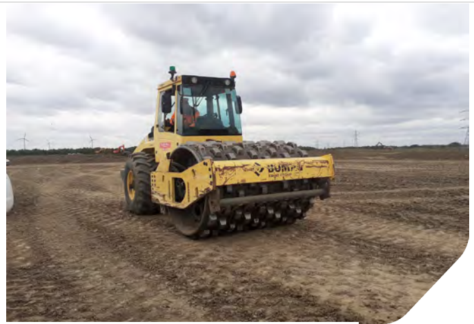
Photo 02: Bomag padfoot roller in Zone 3
