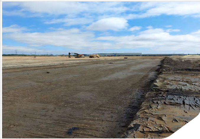
Photo 03: Compacted area in Zone 3
