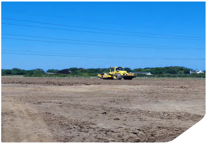
Photo 08: Padfoot roller compacting Zone 3
