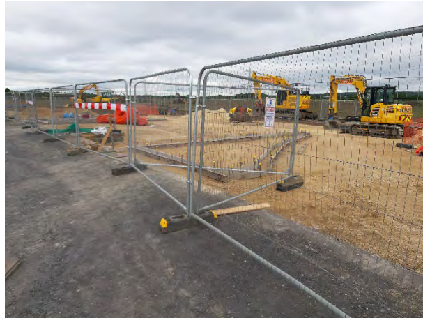
Figure 3. Formation of island within 278 junction works along International Drive.
