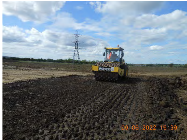
Figure 29. Layer two compaction during passes one and two.
