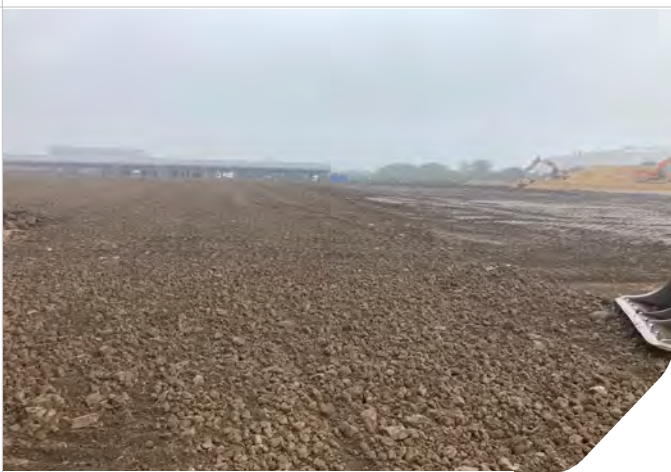
Photo 11: Conditioned clay before rolling in Zone 8
