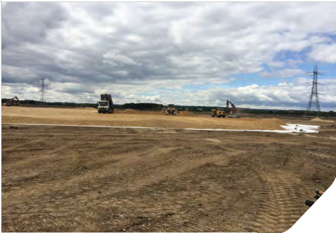
Photo 09: Looking from zone 7 layer 3 across to the Piling matt in Zone 2.
