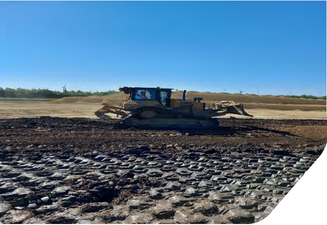
Photo 15: Bulldozer distributing material within Zone 8
