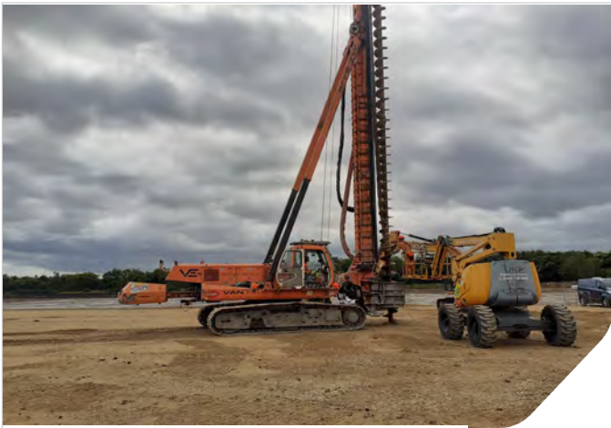
Photo 01: Piling rig preparation in Zone 2
