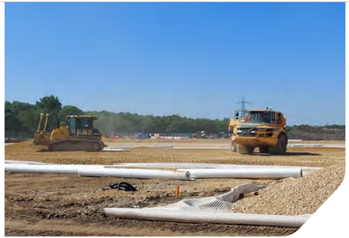
Photo 10: Geomembrane and Type 1 forming piling mat in Zone 5
