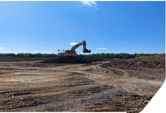
Photo 11: Topsoil bund in Zone 7
