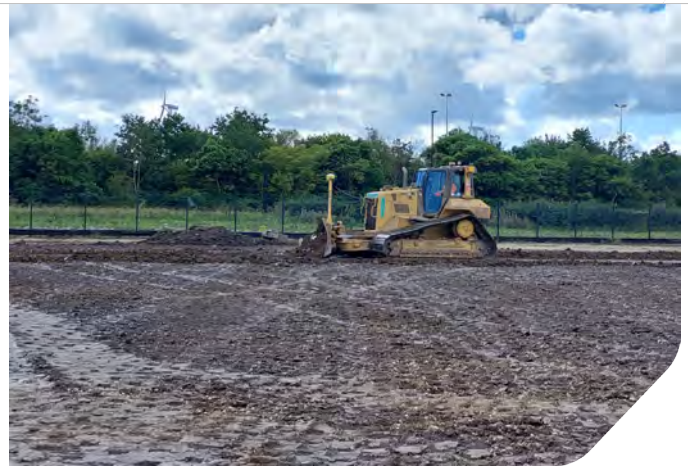
Photo 04: Bulldozer trimming locations of drainage channels within Zone 8
