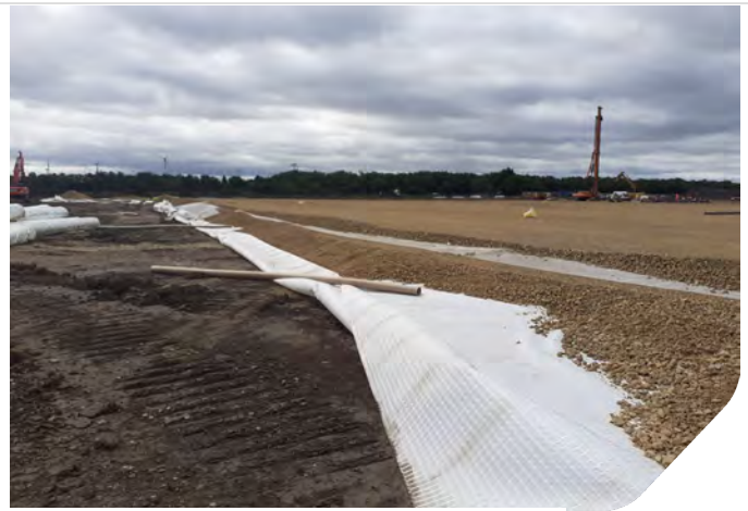
Photo 02: Piling Mat installation
