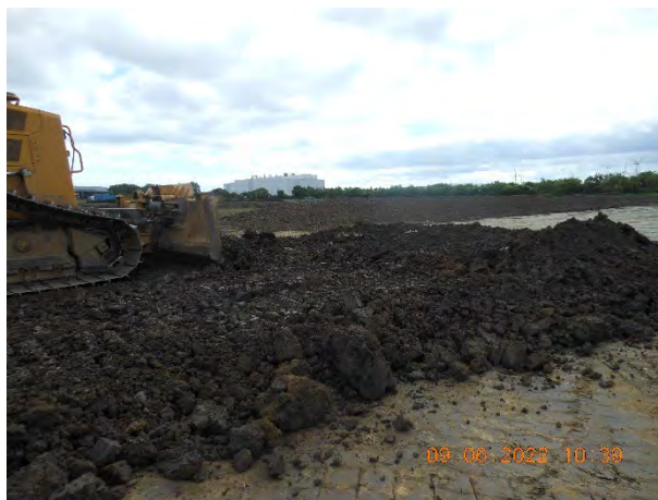
Figure 2. First layer of material being levelled out with dozer.
