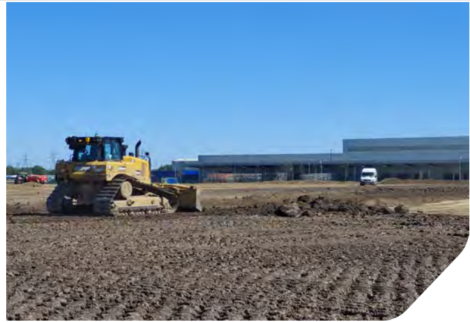
Photo 18: Bulldozer distributing material within Zone 8
