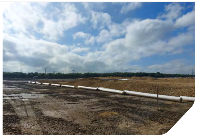
Photo 06: Edge of piling mat within Zone 5
