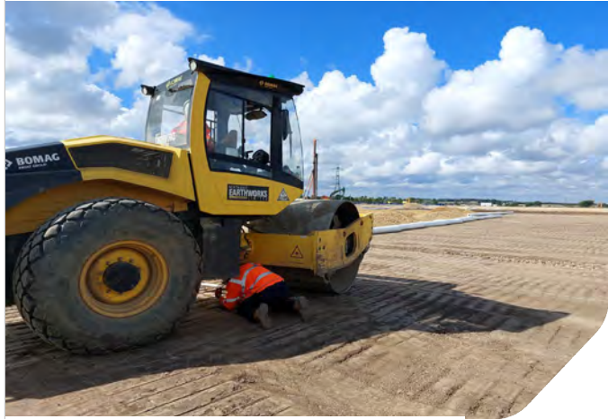
Photo 07: CBR testing in Zone 8
