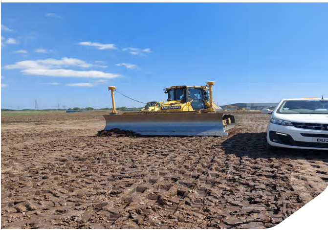
Photo 07: Scraping the dimples off the first testing location pad
