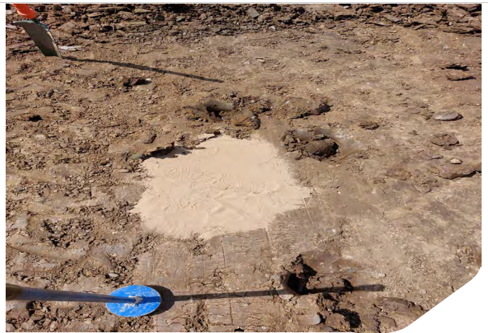
Photo 10: Voids left from core cutter test
