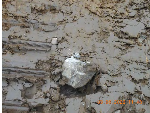
Figure 12. Boulders encountered within fill material.
