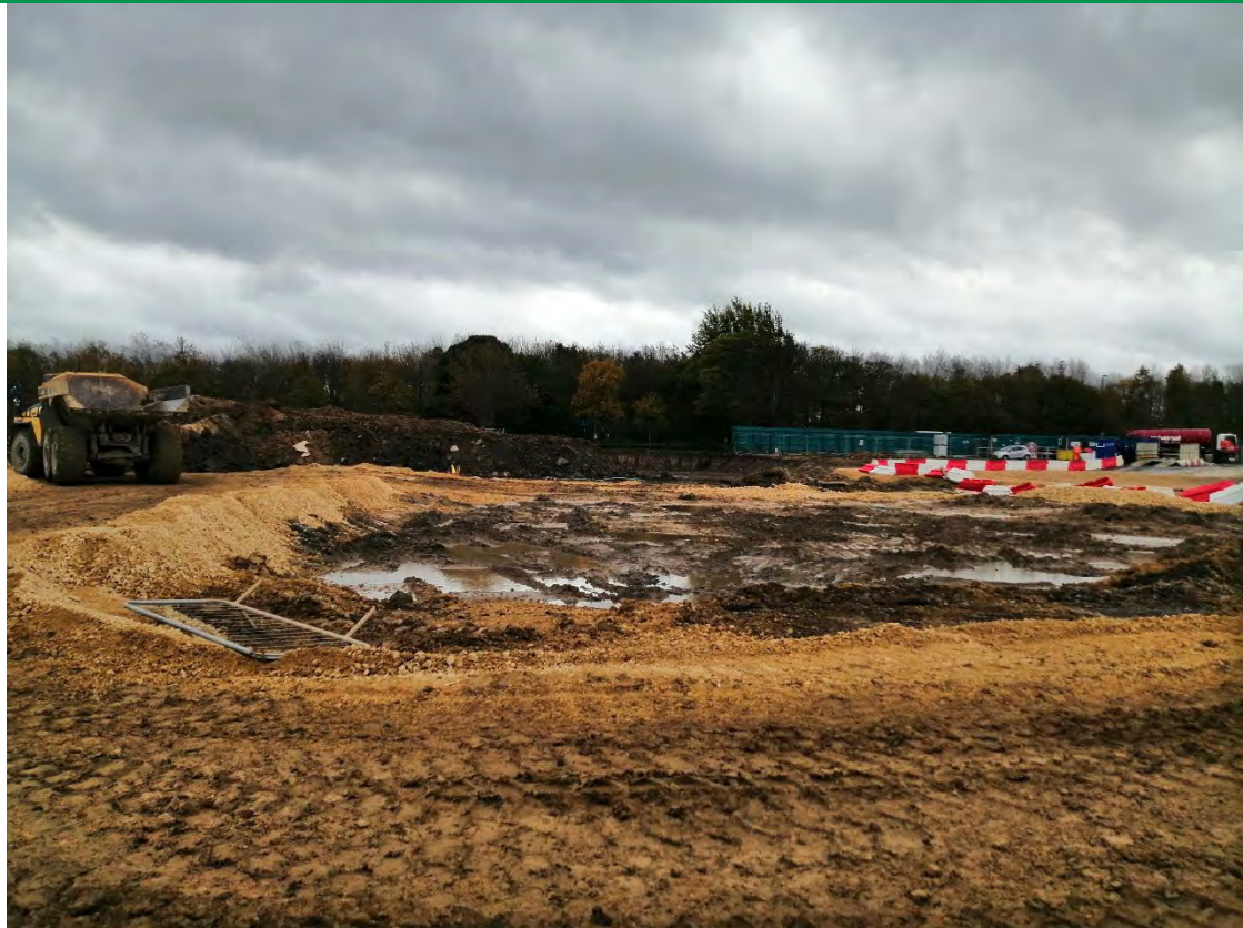
PLATE 4 – LOCALISED SOFT CLAYS ENCOUNTERED WITHIN FOOTPRINT OF FORMER FARM HOUSE
