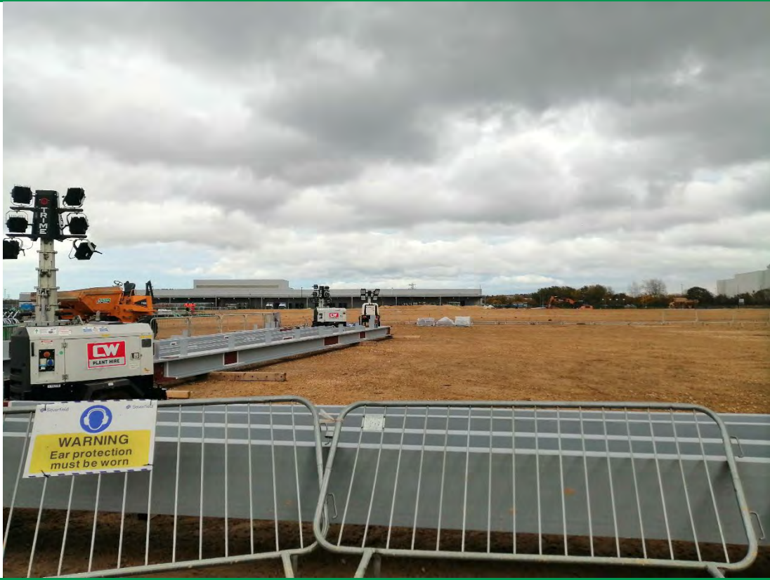
PLATE 5 – STONED-UP LEVELS FOR CONSTRUCTION
