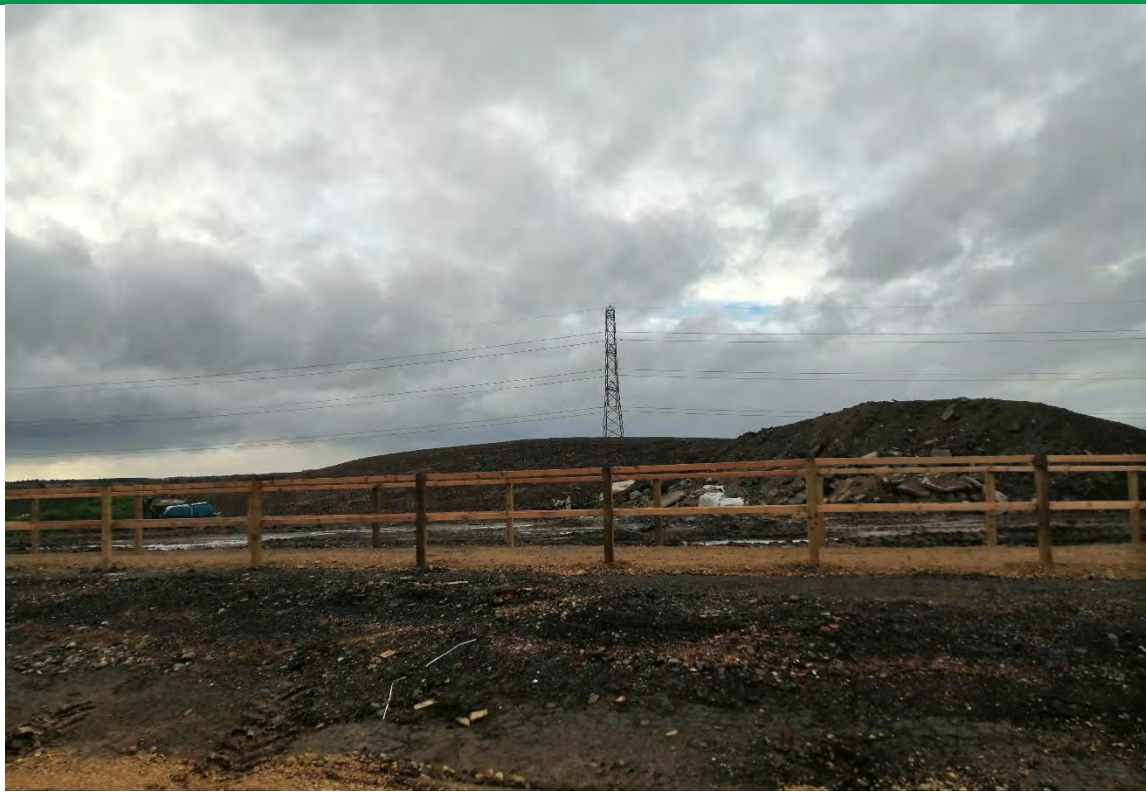
PLATE 3 – CUT SURFACE AND STOCKPILED MATERIALS IN THE SOUTH-WESTERN SITE AREA FOR OFFSITE DISPOSAL
