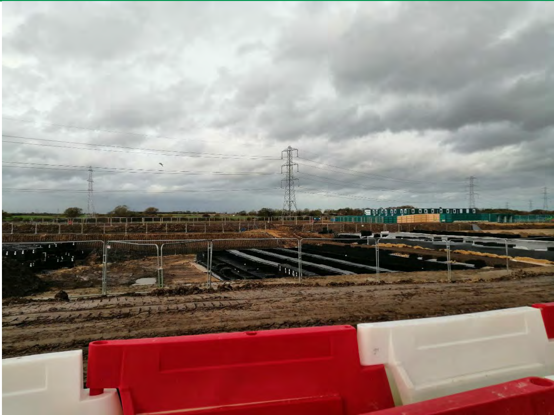
PLATE 1 – INSTALLATION OF THE CRATE STORAGE
