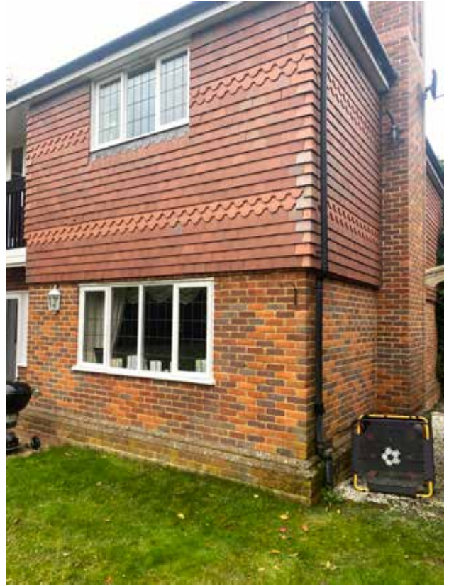
View from SW corner
