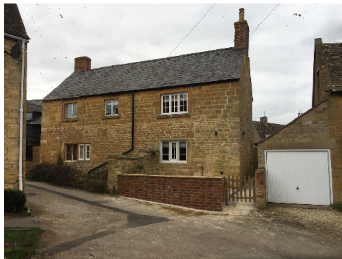
The demarcation between Millbank Cottage and Primrose Cottage is shown on drawing 24180
