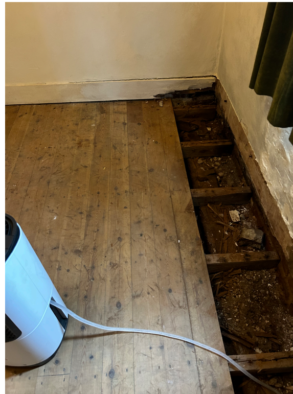
Modern floor boards over modern joists.
