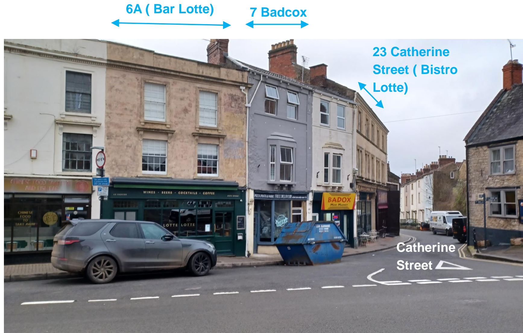
Fig 2 : External elevation of 6A and 7 Badcox – No external changes proposed (photo taken from the corner of Weymouth Road and Badcox
