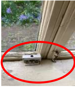
Excessive gapping when closed
