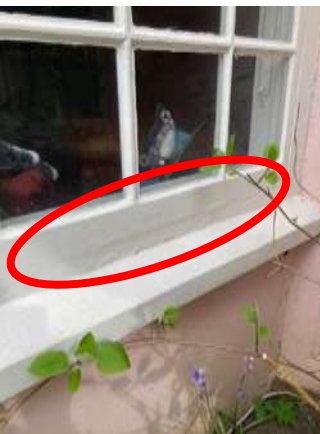
Repeatedly filled external frame & sill
