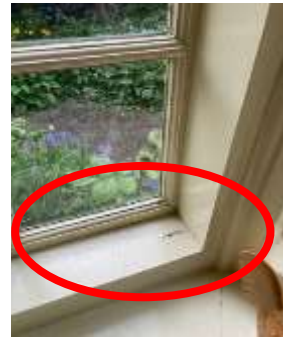
Frame deterioration
