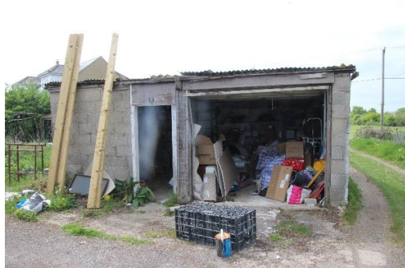
6. The double garage and workshop (4)
