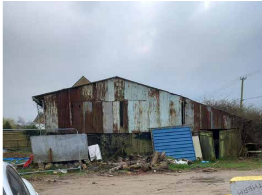
Outbuilding proposed for demolition.
