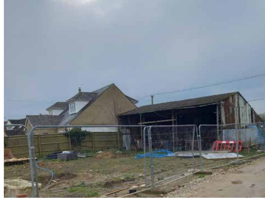
Outbuilding proposed for demolition.
