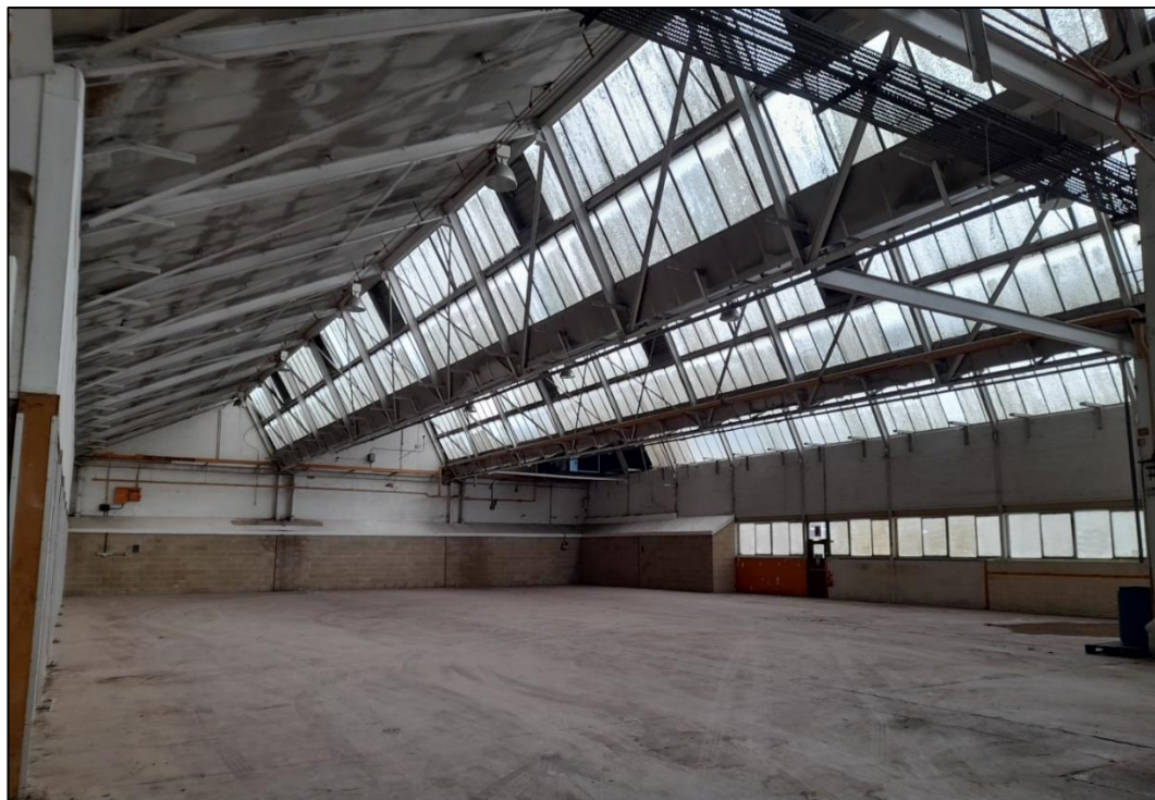
Photograph 6 and 7: Internal views of mezzanine office and main warehouse of B1
