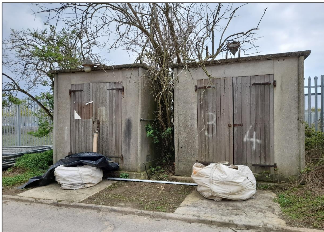
Photograph 1: Concrete sheds that could not be fully accessed.
