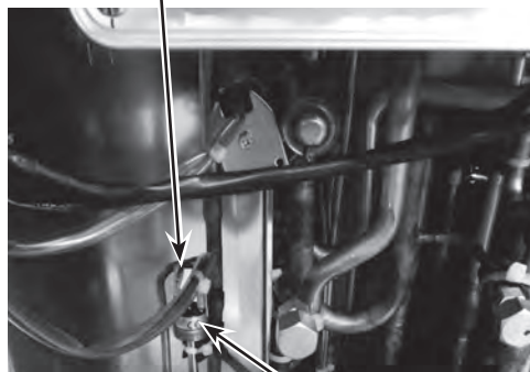
High pressure switch (63H)
