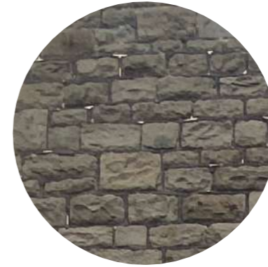
Example of walls
