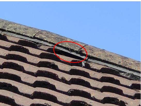
Plate 15: Gaps at the eaves around the bay window on the south-east elevation of the church
