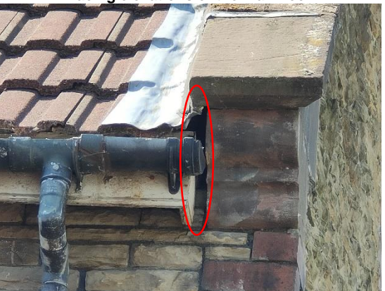
Plate 16: Gaps at the eaves on the south-west facing elevation of the main roof
