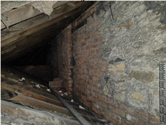
Plate 13: Gaps beneath ridge tiles
