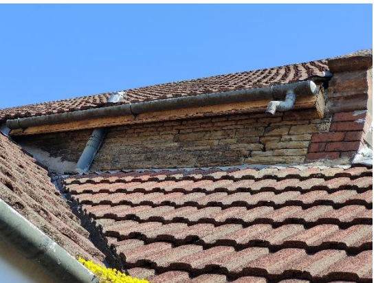
Plate 16: Gaps at the eaves on the south-west facing elevation of the main roof
