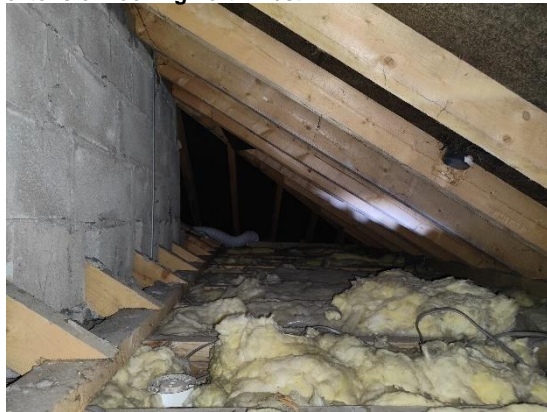
Plate 14: Gaps at the eaves on north and south facing elevations of the main roof
