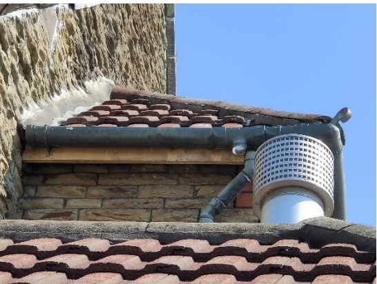
Plate 15: Gaps at the eaves around the bay window on the south-east elevation of the church
