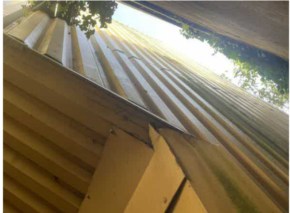
Photo 32: Western Side of B1d
