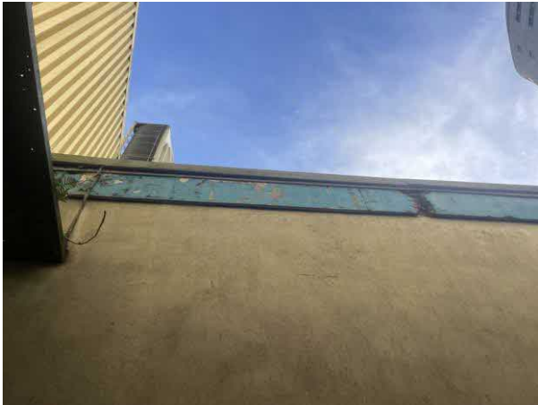
Photo 39: Broken and Raised Fascia and Raised Metal Trim on Northern Side of B2
