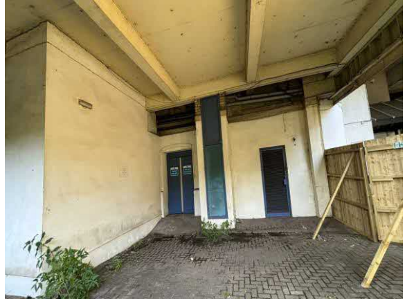
Photo 2: Southern Rear of B1a
