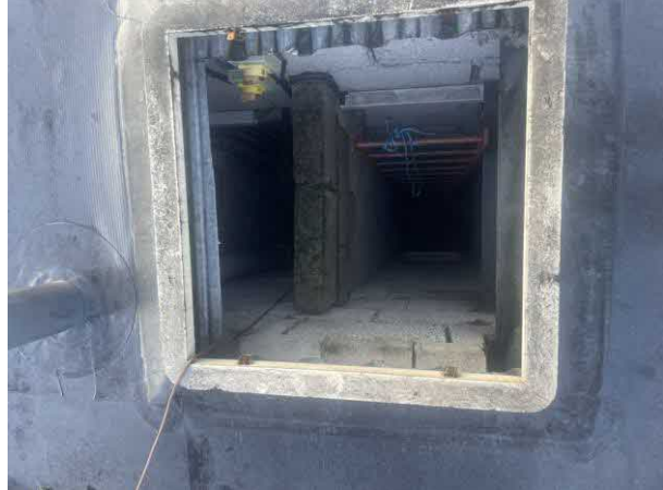
Photo 38: Open Access Point to the Roof of B1b
