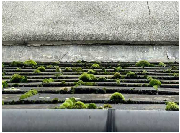
Photo 22: Raised Roof Tiles on Southern Side of B1c
