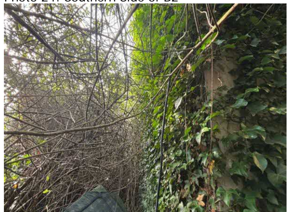
Photo 24: Southern Side of B2
