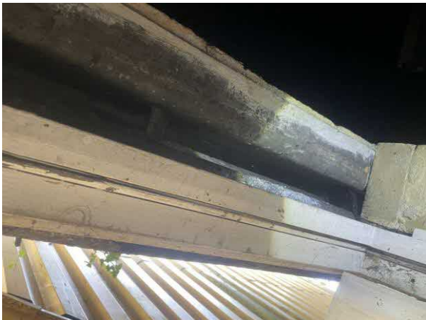
Photo 50: Internal Gap Above the Door Frame of B2
