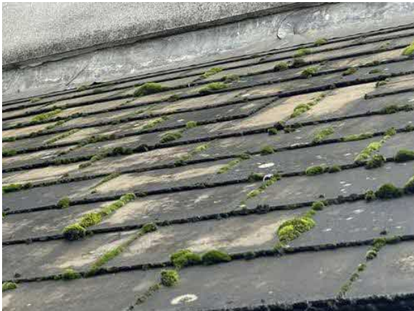
Photo 21: Missing and Raised Roof Tiles on Southern Side of B1c
