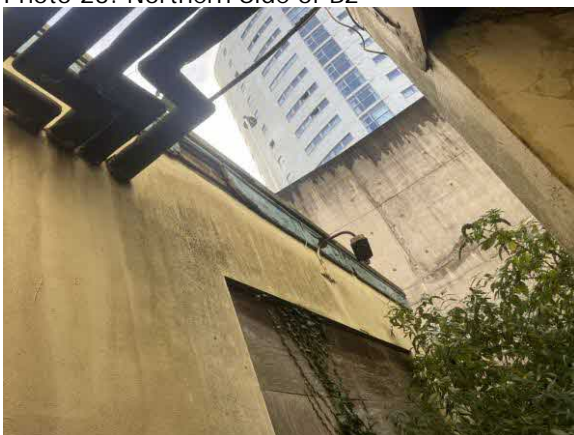
Photo 23: Northern Side of B2
