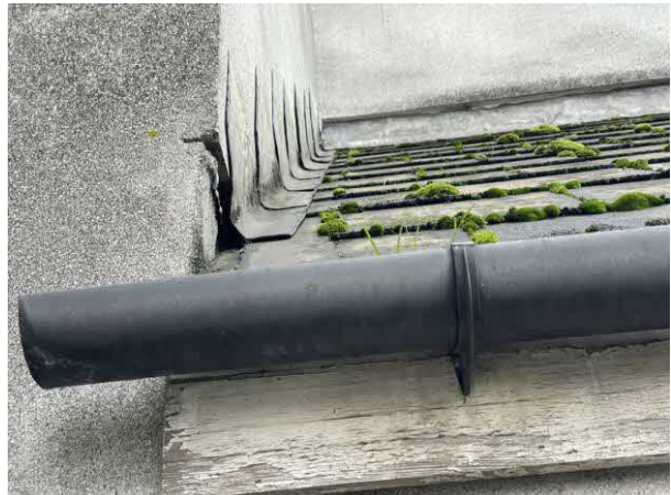
Photo 22: Raised Roof Tiles on Southern Side of B1c
