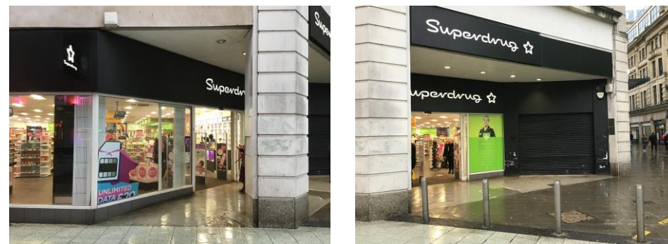
Figure 4 : Existing shop front and entrance doors
