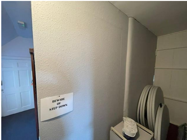
View of rear wing back hall
