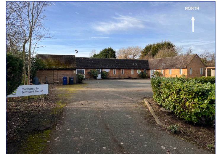
Office building viewed from entrance drive 2022
