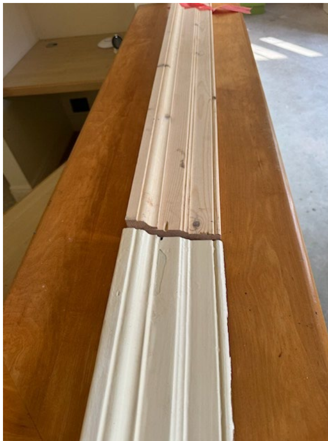
Image 1 – Sample Architrave Repair
