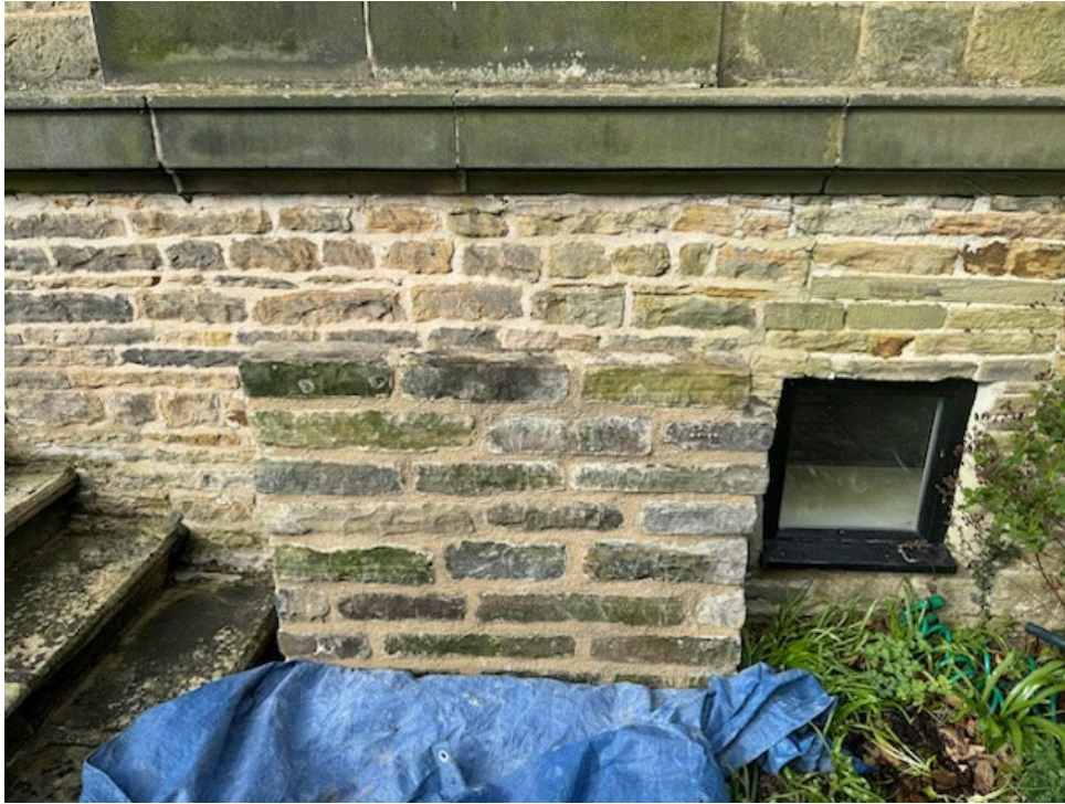
Image 2 – Sample Lime Mortar Panel
