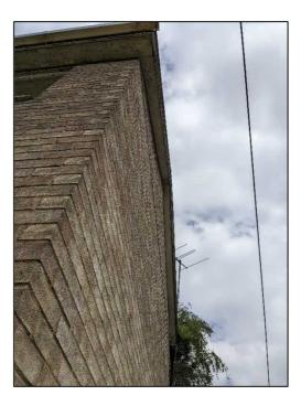
3.3.5. Soffits are present on all sides of the building and they are in good condition, and are fitted flush to the walls with no gaps behind, offering no access opportunities for bats.
