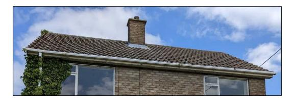
3.3.4. The mortar along the gables is in excellent condition, with none missing to allow bats access into the building or below the tiles.
