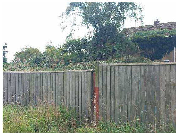
Photograph 8: View of the rear of the building and outhouse.
