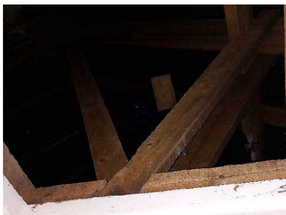
Photograph 13: View of the roof timbers (1)
