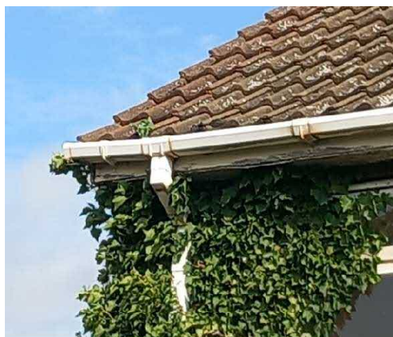
Photograph 5: View of front gutter and Exterior roof timbers
