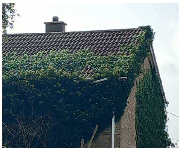
Photograph 6: View of rear gutter
