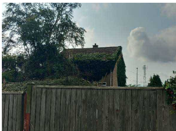
Photograph 3: Rear View of Building
