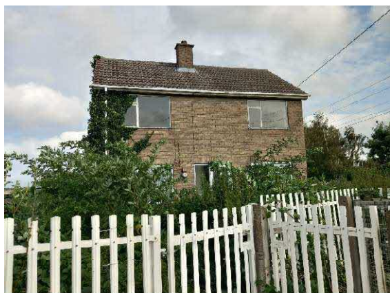
Photograph 1: Front View of Building (1)
