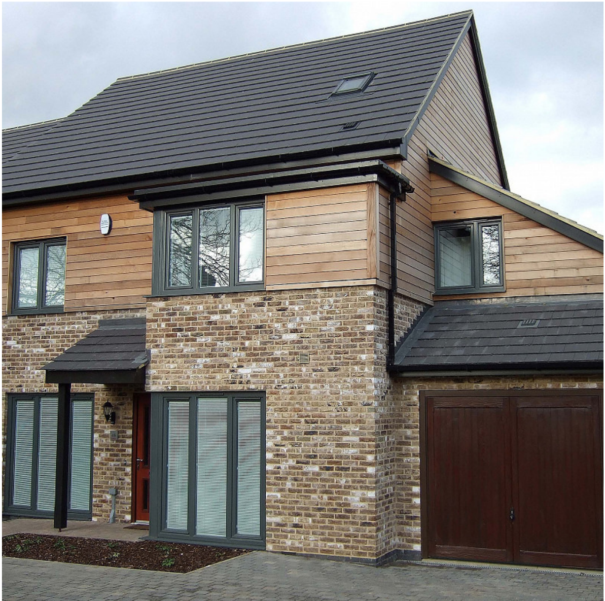
WALL: LONDON WEATHERED YELLOW STOCK BRICK (TBS) - COMBINED WITH NATURALLY AGING CEDAR CLADDING.
