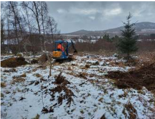
Photo 2 Showing digging of Test Pit
