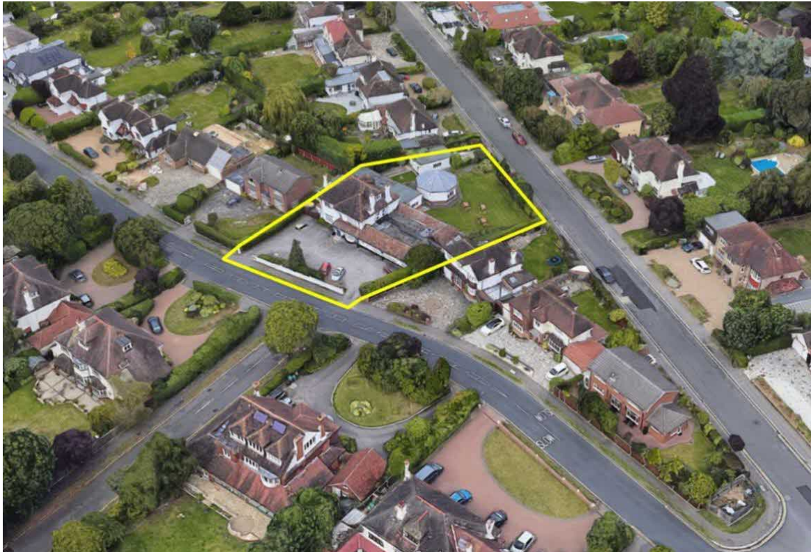
Figure 1: Aerial view of the site, outlined approx. in yellow
