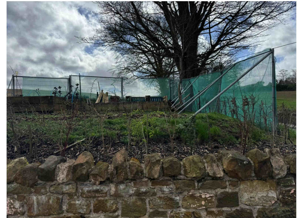
Photo 2: existing temporary metal and wire wind break fence
