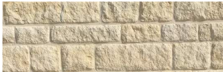
Coursed Rubble Walling
