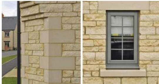
Clipsham Ashlar with Coursed Rubble Walling
