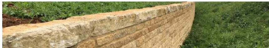
Coursed Rubble Walling
