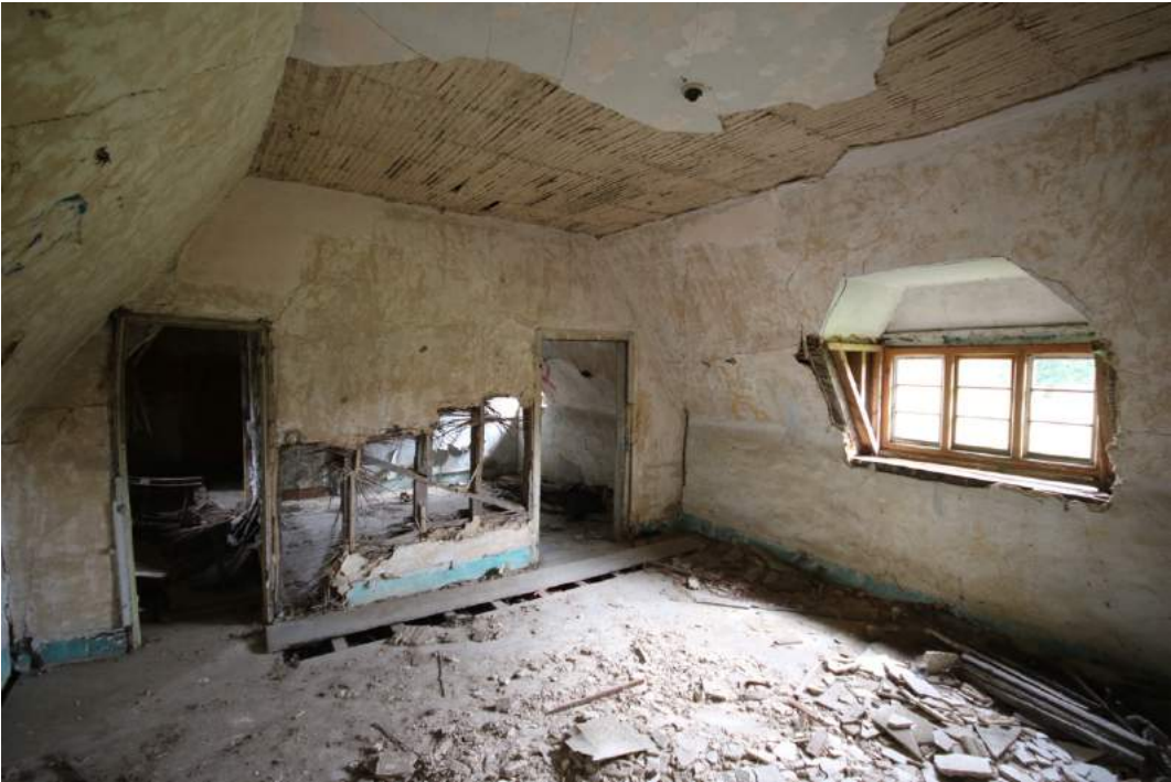
Main bedroom with single board raised for inspection. All boards are to be taken up to facilitate repair and M&E installation.
