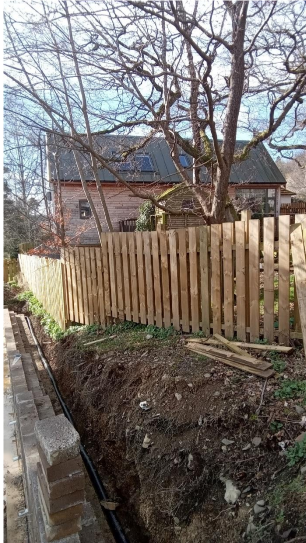
ELM (3716) DETAIL EXCAVATION IN ROOT ZONE
