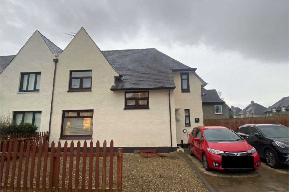
Fig. 1: View of North Elevation.
