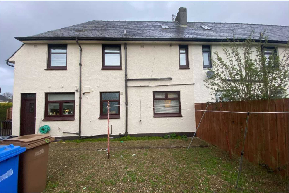
Fig 2: View of South Elevation.
