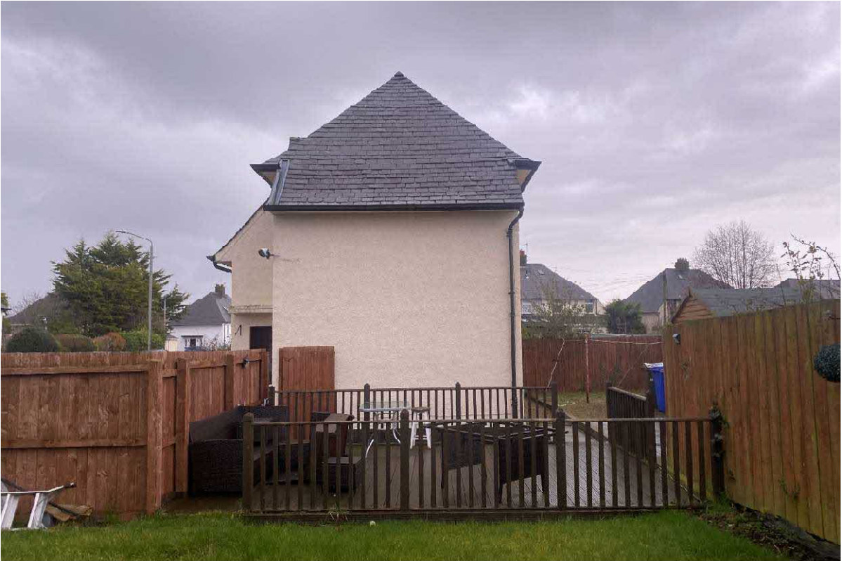
Fig. 6: View of East Elevation.
