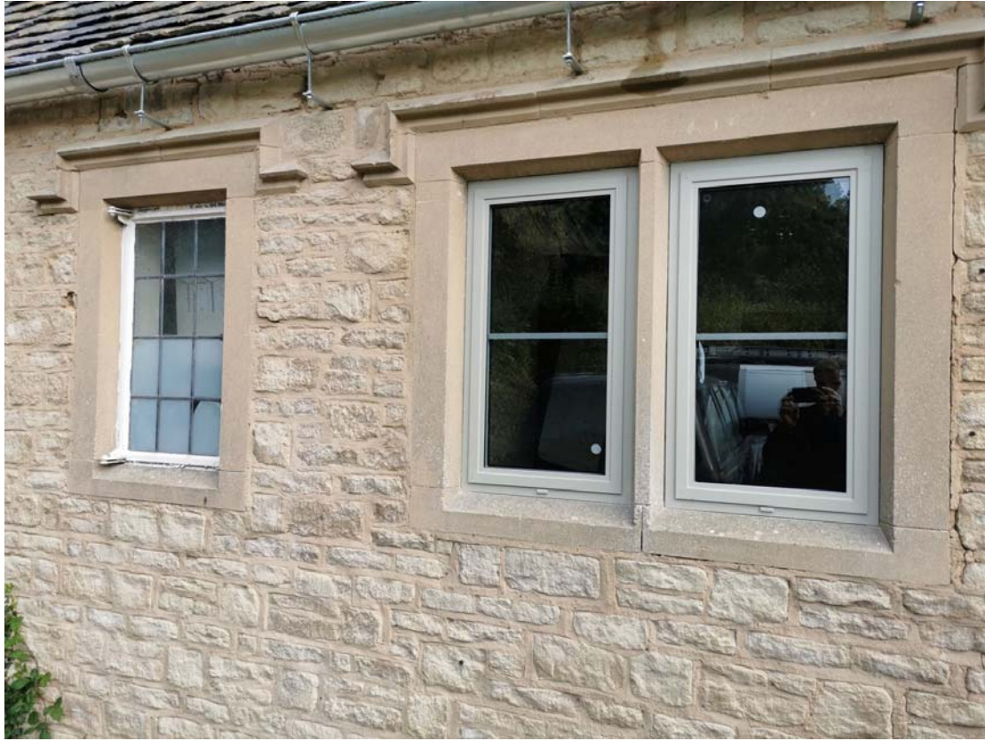
Above: example of the proposed windows (right) and an existing window (left)
