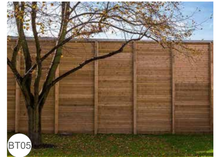
Acoustic Fence Height: 3m Material: Wood
