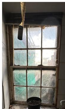
All are single glazed, timbers are noted to be rotten internally and externally. Large sections of timbers have fallen away and paint is peeling away to the majority.
